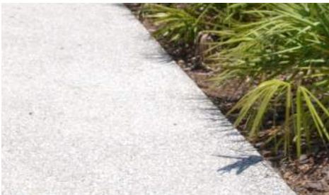
EXPOSED AGGREGATE CONCRETE
