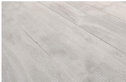
BOARD FORMED / STAMPED CONCRETE
