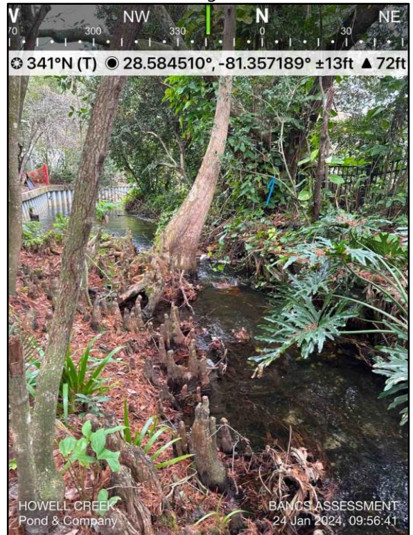
Photograph 72: BEHI = Moderate, NBS = Moderate; ~Sta. 13+50.
