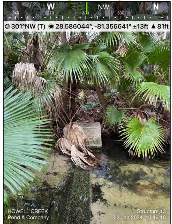
Photograph 32: Grade Control Wier downstream of Structure 13 (Priority 4)
