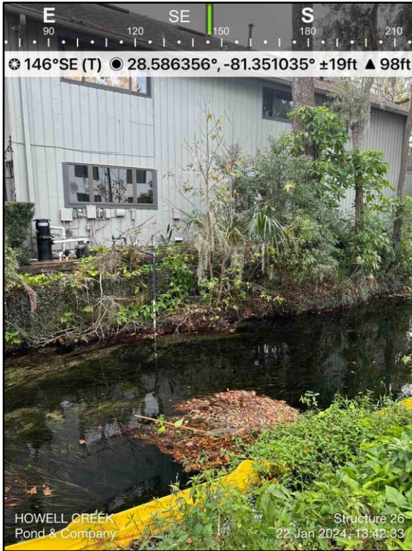
Photograph 61: Structure 26; Wooden Retaining Wall (Priority 4)
