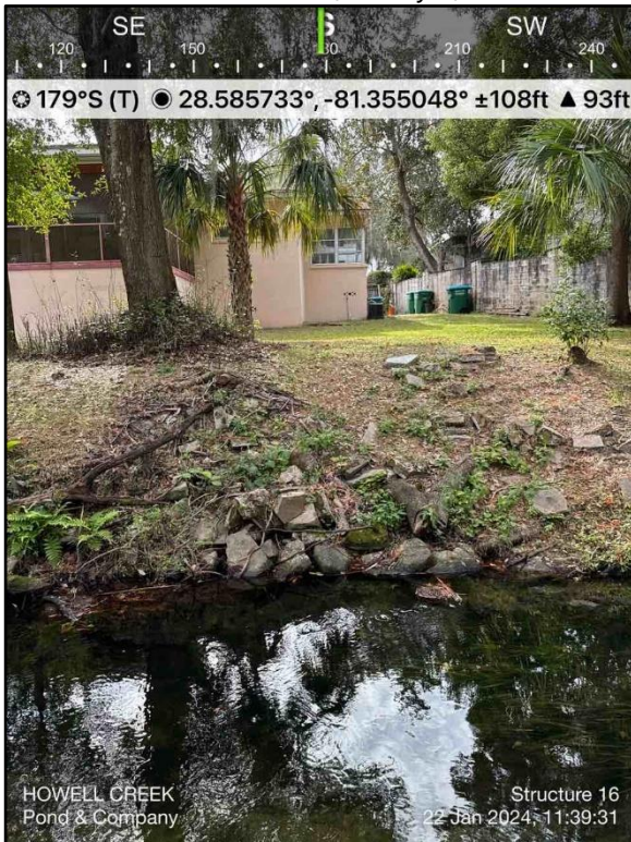
Photograph 39: Structure 16; Rock Streambank Protection & Concrete Bag Wall (Priority 0)
