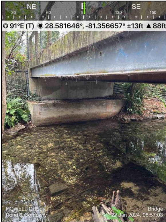
Photograph 5: Bridge Crossing of Upstream Reach of Howell Creek
