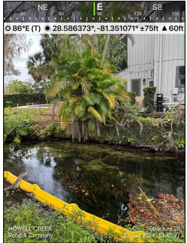
Photograph 62: Structure 26; Wooden Retaining Wall (Priority 4)
