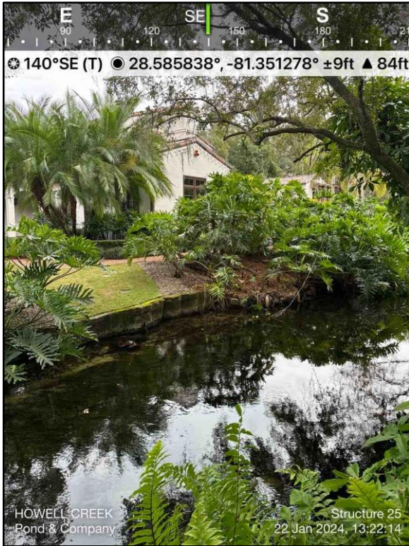
Photograph 57: Structure 25; Concrete and Wooden Retaining Wall (Priority 0)
