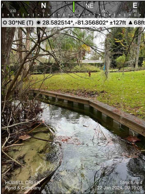
Photograph 9: Structure 4; Sheet Pile Wooden Capped Retaining Wall (Priority 3)
