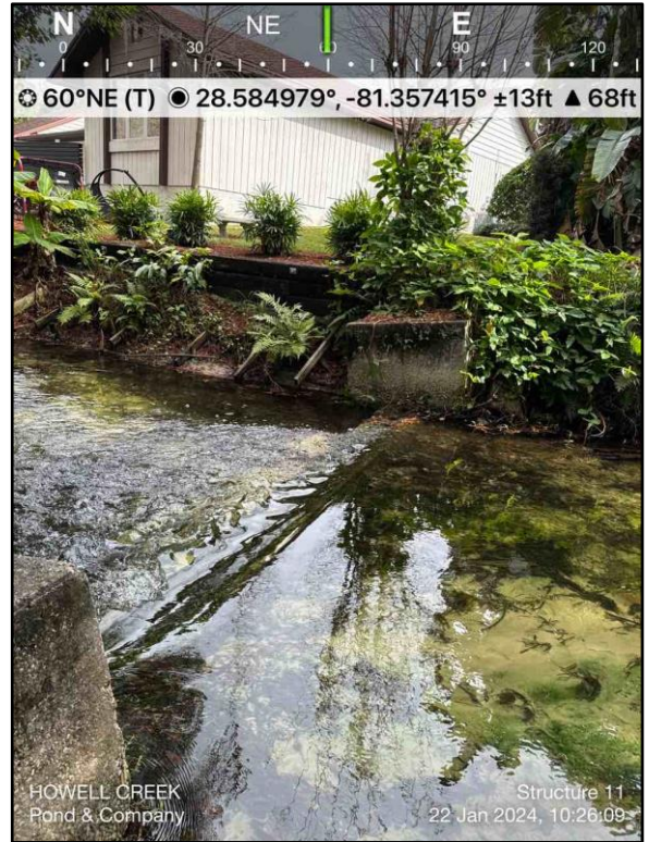
Photograph 26: Structure 11; Grade Control Weir and Adjacent Wooden Retaining Wall (Priority 4)
