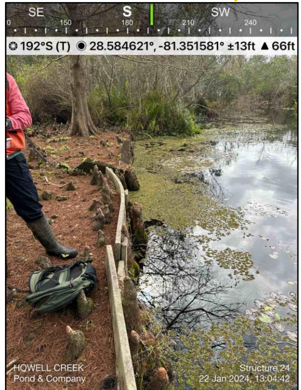
Photograph 56: Structure 24; Wooden/Composite Retaining Wall (Priority 2)
