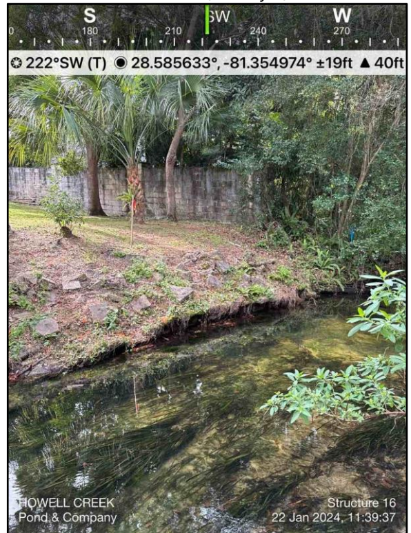
Photograph 40: Structure 16; Rock Streambank Protection & Concrete Bag Wall (Priority 0)
