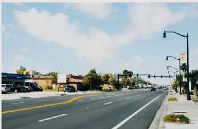
A stretch of Fairbanks Avenue should have a much different look by the end of 2019. These photos from the city show the before (top) and after (bottom).
