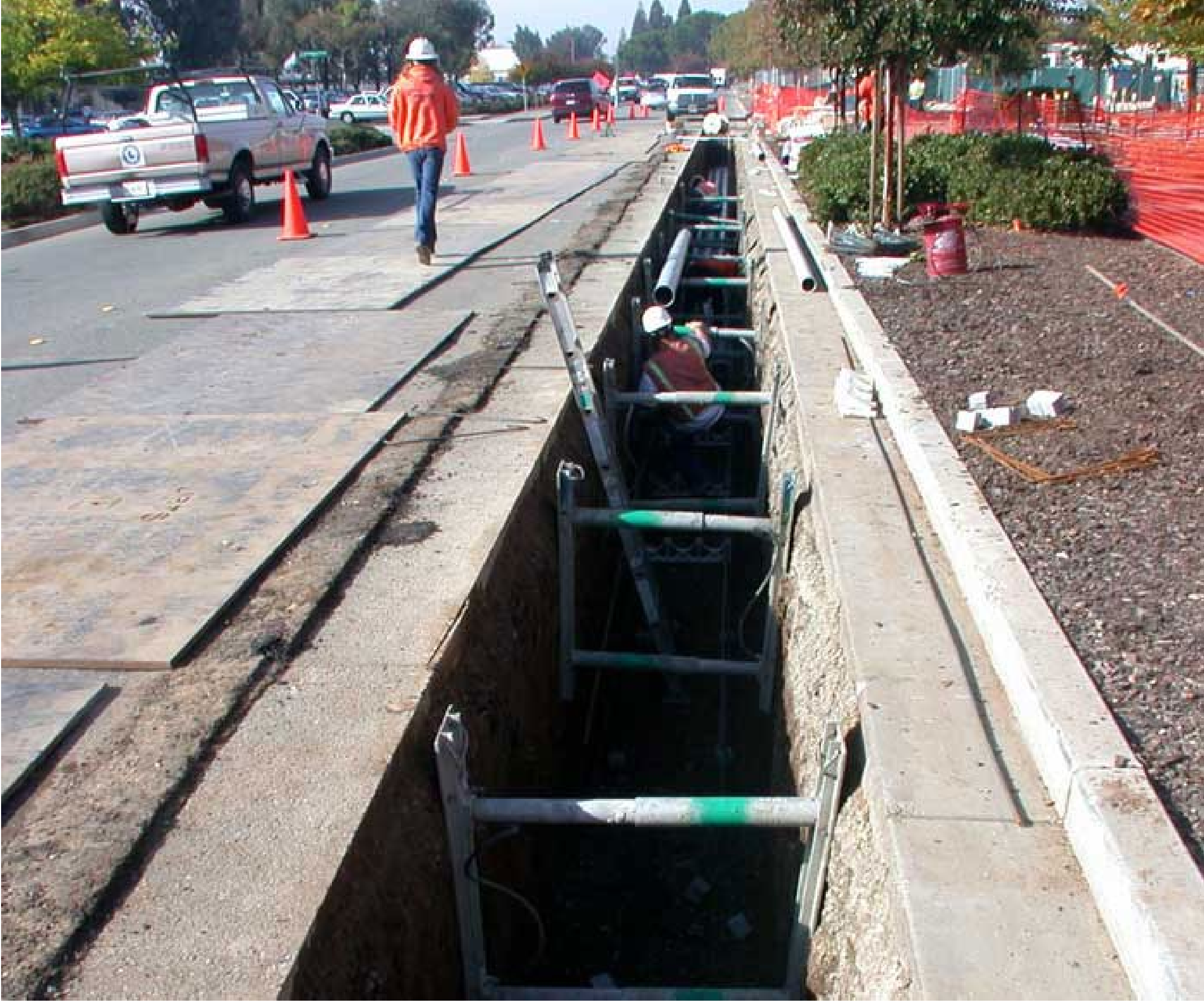
Shallow duct bank along curb. Concrete vertical barriers may be installed between the curb and sidewalk in some areas.
