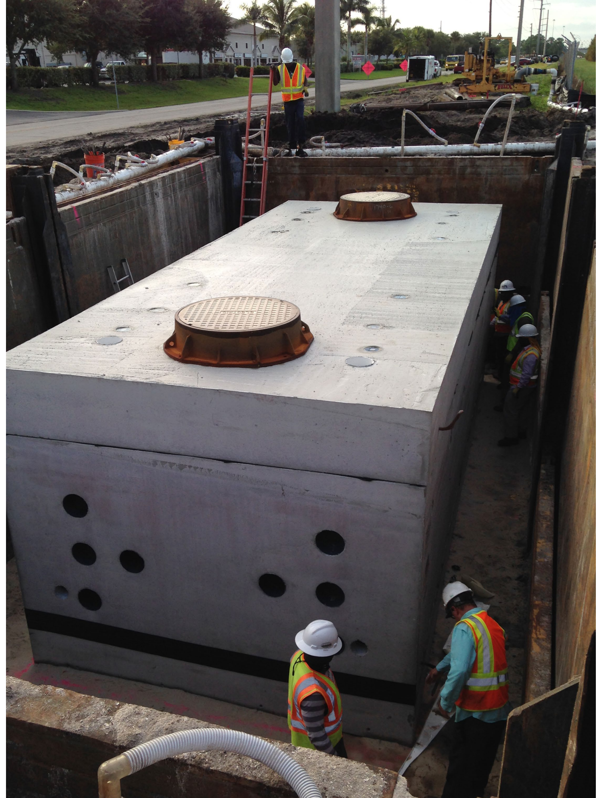
Manhole structures
