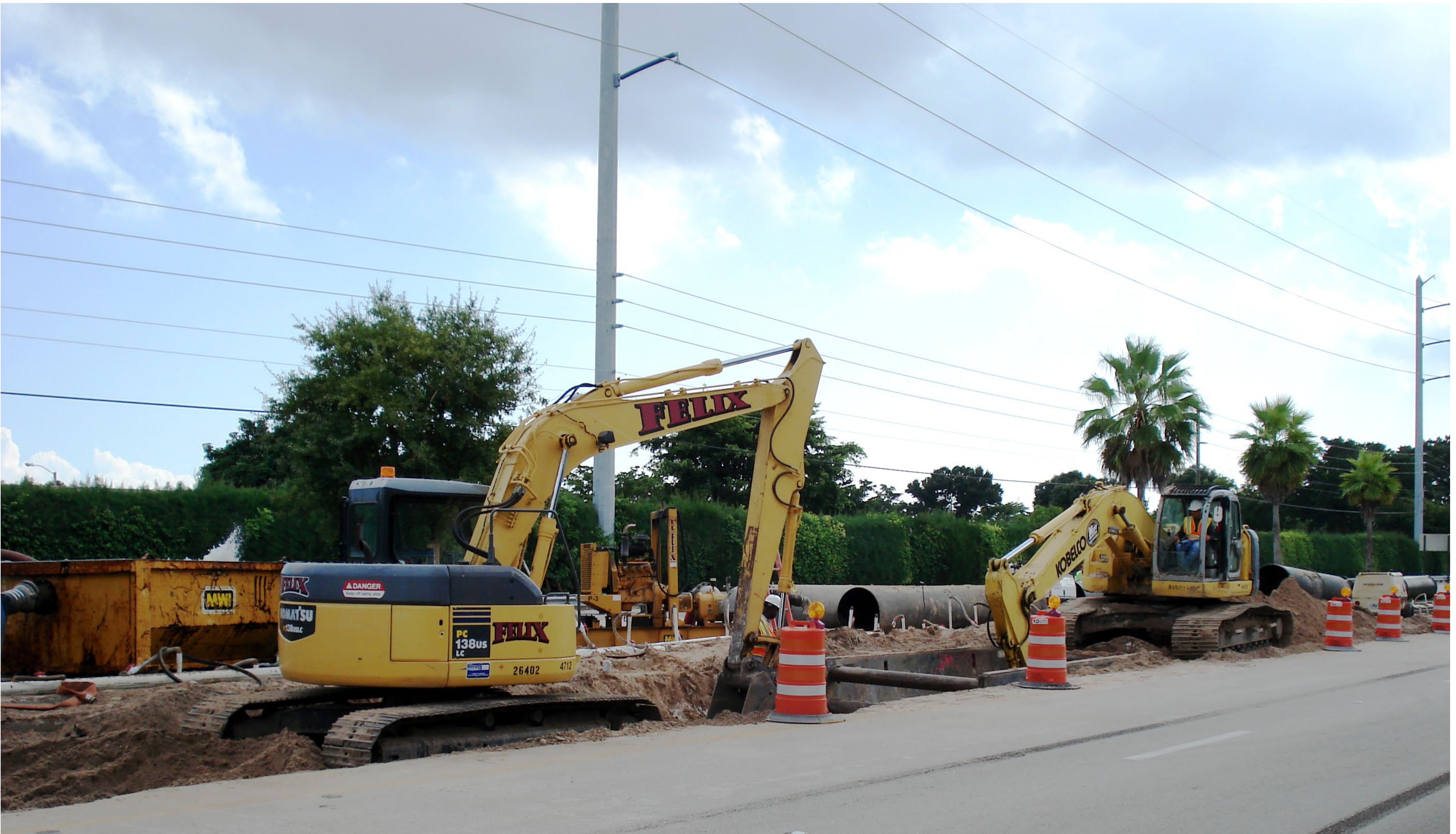
Excavation in roadway
