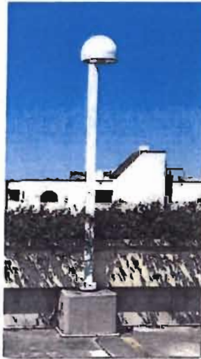
Low height poles and fixtures reduce the off-site rooftop visibility of rooftop lighting. Directional fixtures reduce light spread and meet "dark sky" requirements.
