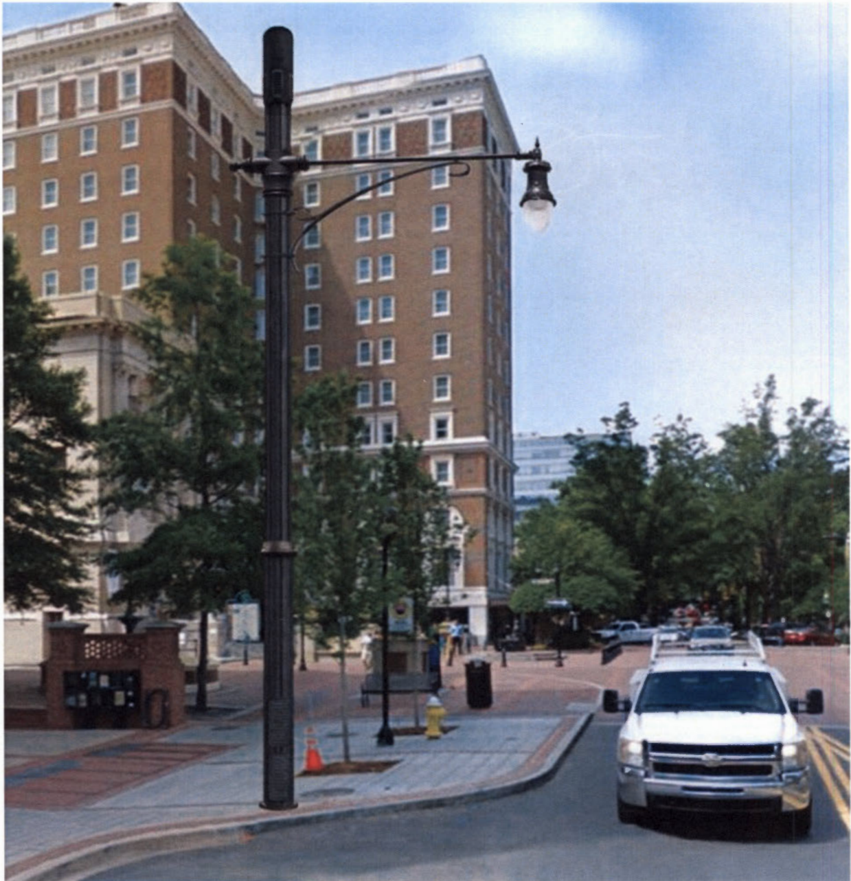
Exhibit 1. Simulated fluted pole to be manufactured by Nepsa with capacity for two internal, collocated wireless antennas. Decorative mast arm and down lighting luminaire by Sternberg Lighting, the manufacturer of the City's decorative lights. This would be an acceptable design with an arm that matched the design of the City's existing decorative lights; however, the pole's location, mere inches from the curb, would violate the 8 foot clear space requirement from the curb or edge of pavement. The light pole design may also be acceptable on certain streets with double mast arms matching the design of the City's existing decorative lights and down lighting luminaires by Sternberg mirroring one other.
