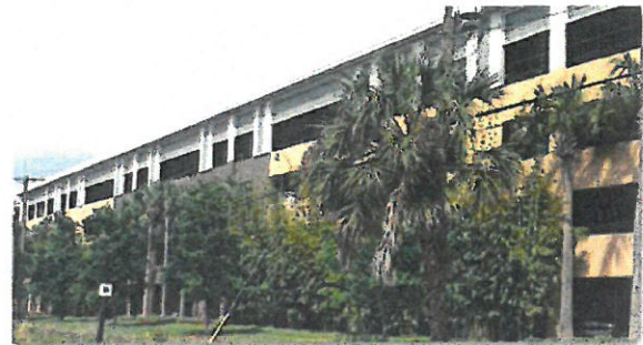
Significant landscape screening works to screen a very long wall façade of this parking garage
