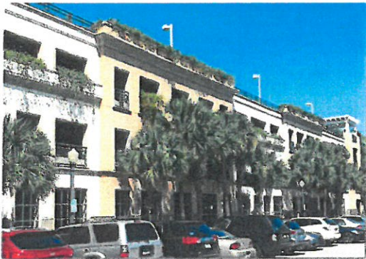
Landscaping is one element in attractive look of the Sun Trust garage.
