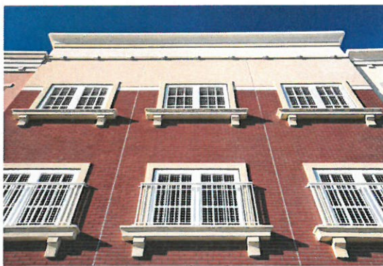
Exceptional window/opening treatments combine with cornice and color.
