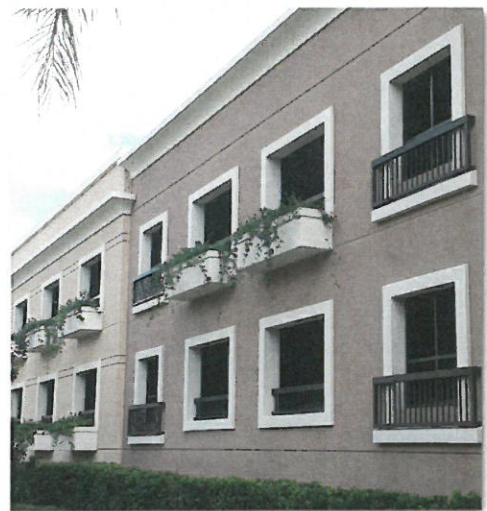
Planter boxes, window grills, protruded balconies and window framing provide the appearance of windows.
