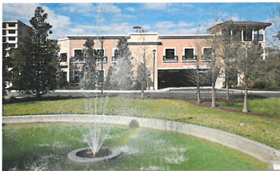
WP Towers garage with cornice, articulation, stair tower, window fenestration, planter boxes and opening framing details combine successfully.
