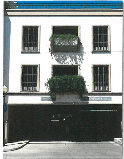
Cornice, expression lines, window boxes and window grills.
