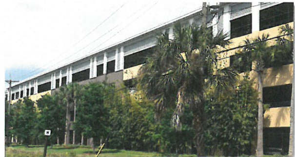
Significant landscape screening works to screen a very long wall façade of this parking garage
