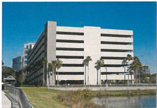
Example of precast concrete panels with minimal interest
