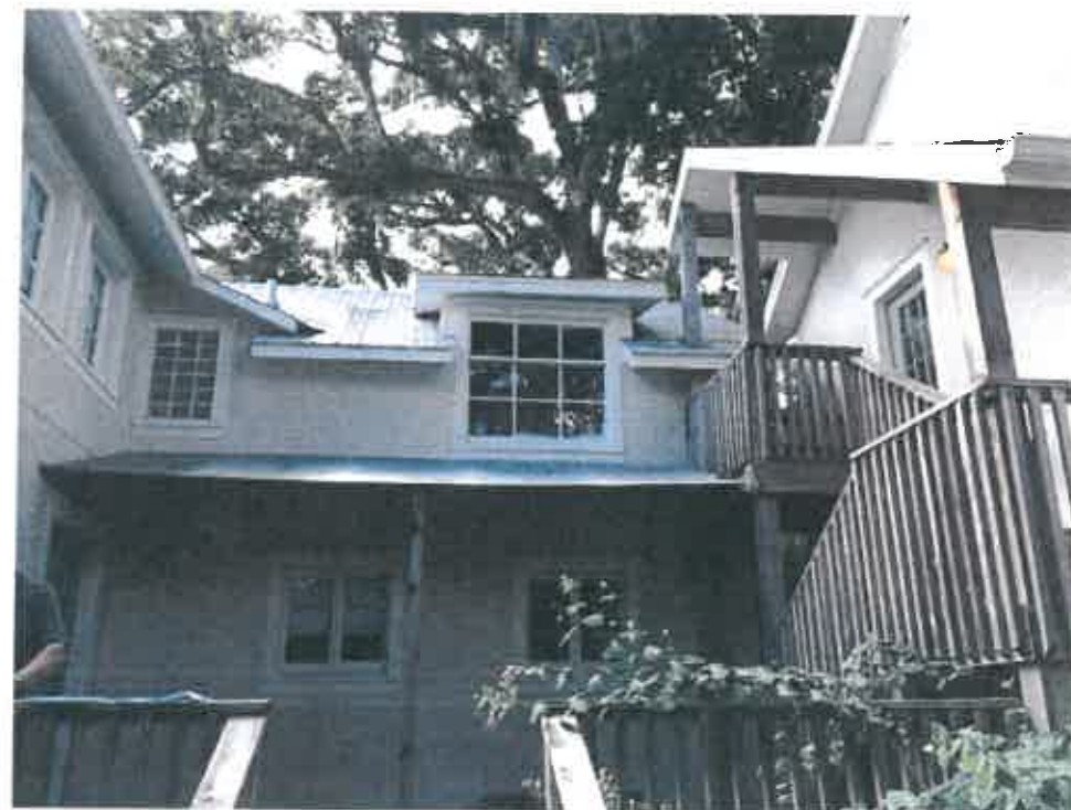
Existing House: view from East (rear yard)
