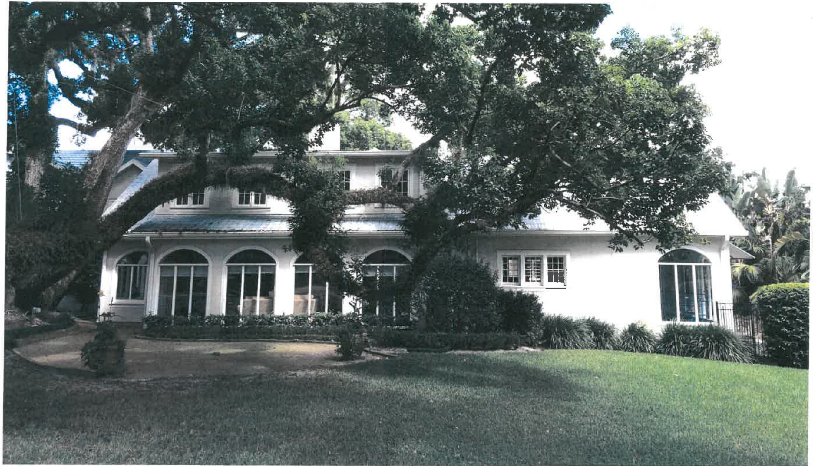
Existing House: view from Greentree Drive (West)
