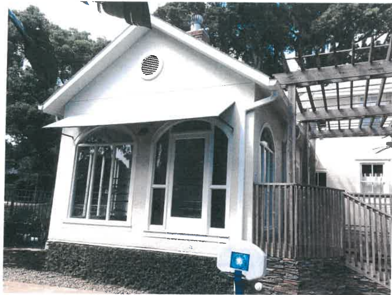
Existing House: view from South
