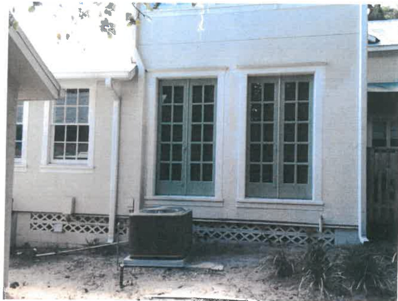
Existing House: view from East (rear yard)
