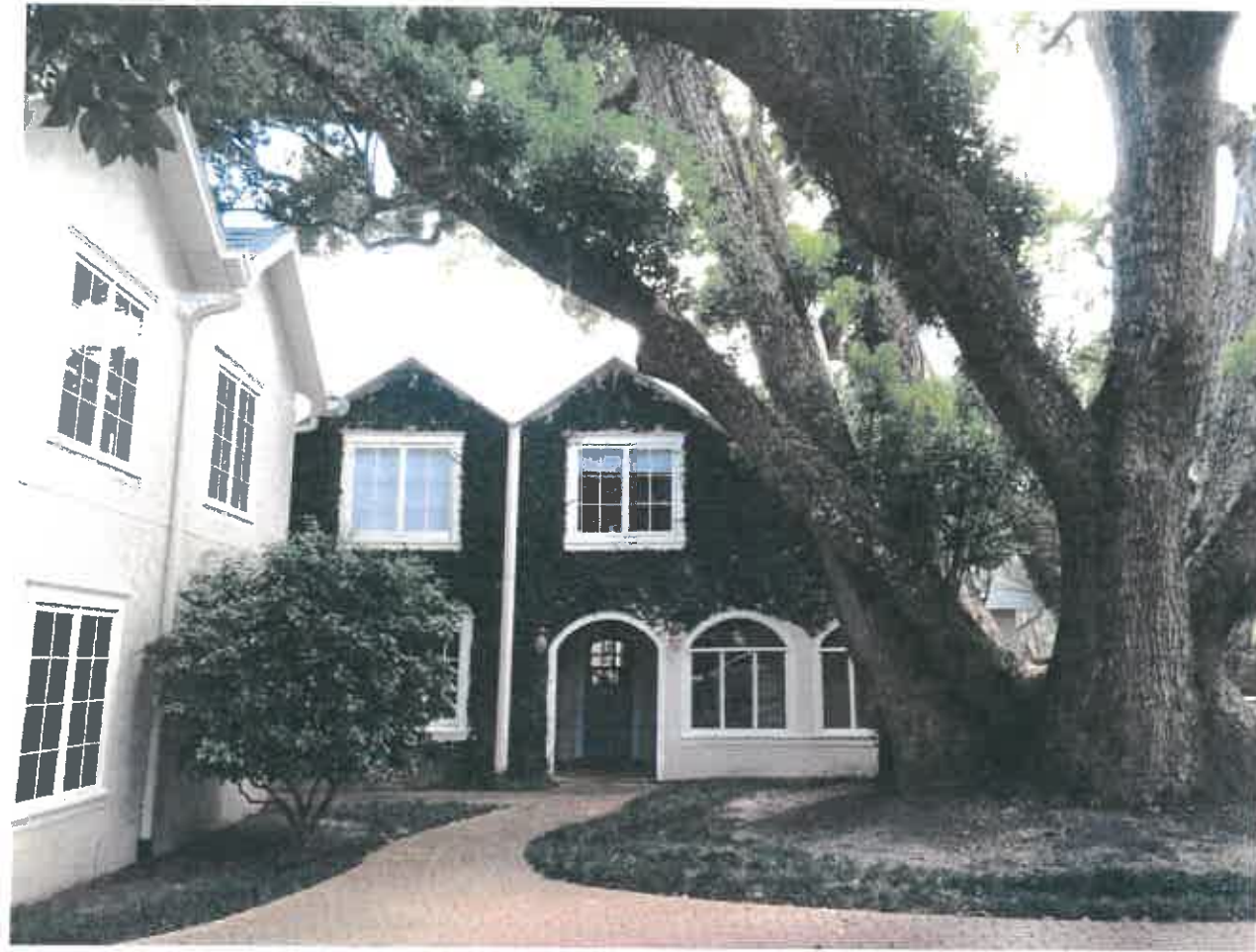
Existing House: view from North)
