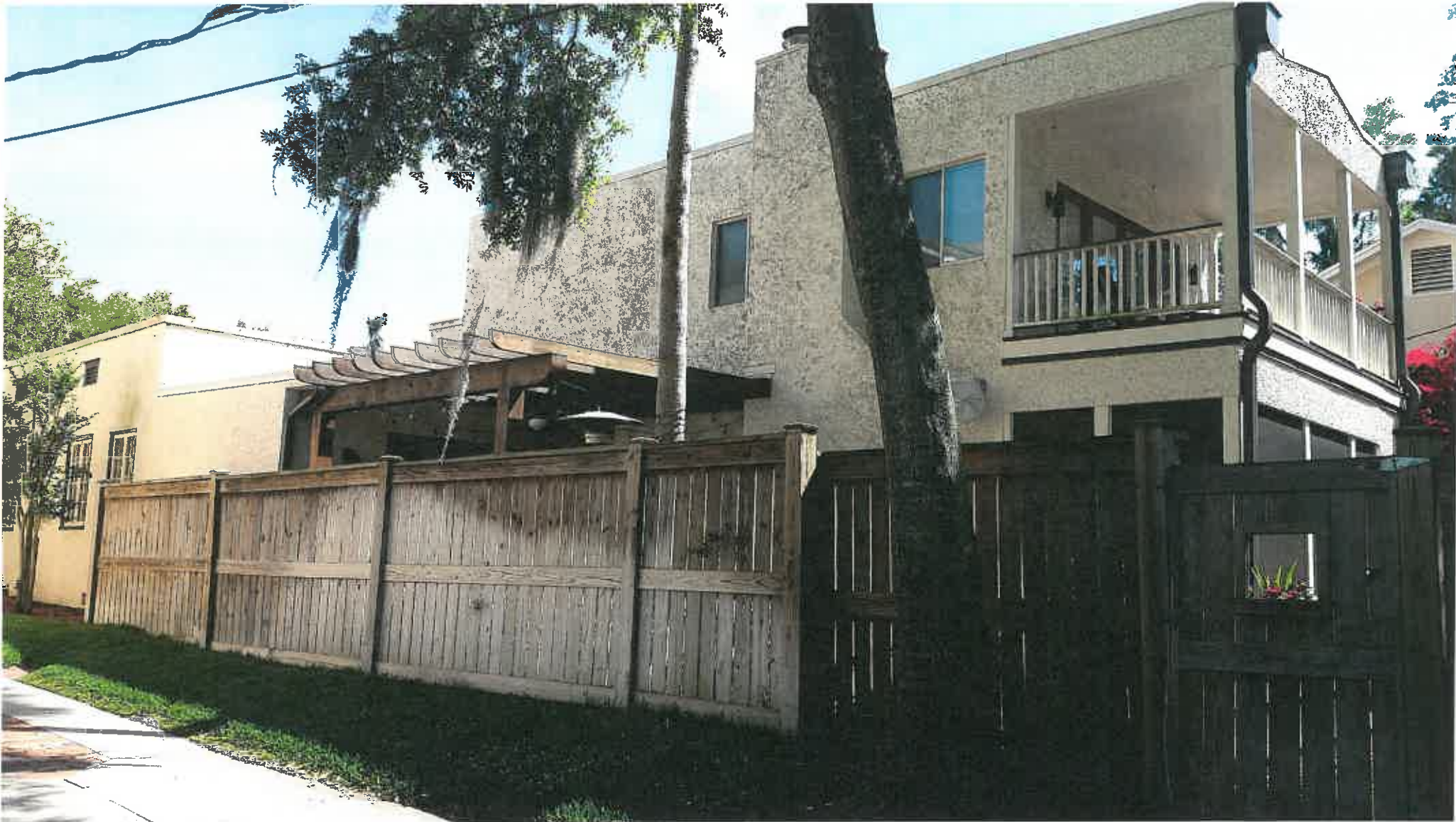
WEST SIDE ELEVATION FROM REAR
