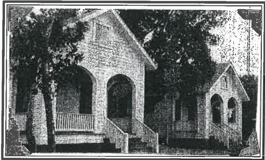
HISTORICAL PHOTO: VIEW FROM SOUTHWEST
