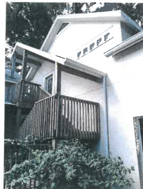
Accessory Bldg: view from South
