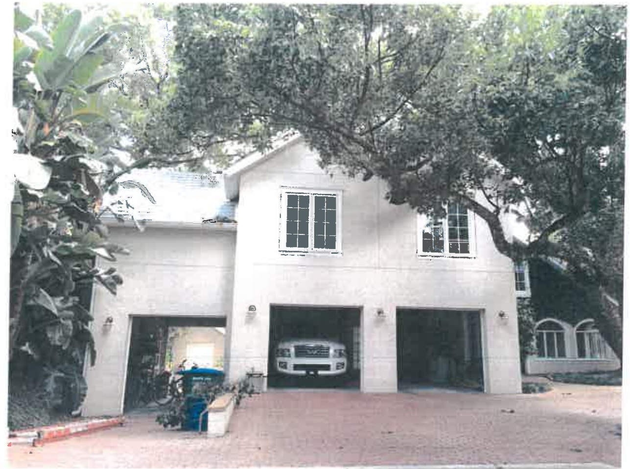
Existing House: view from North
