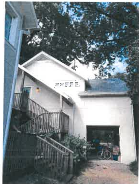
Accessory Bldg: view from South
