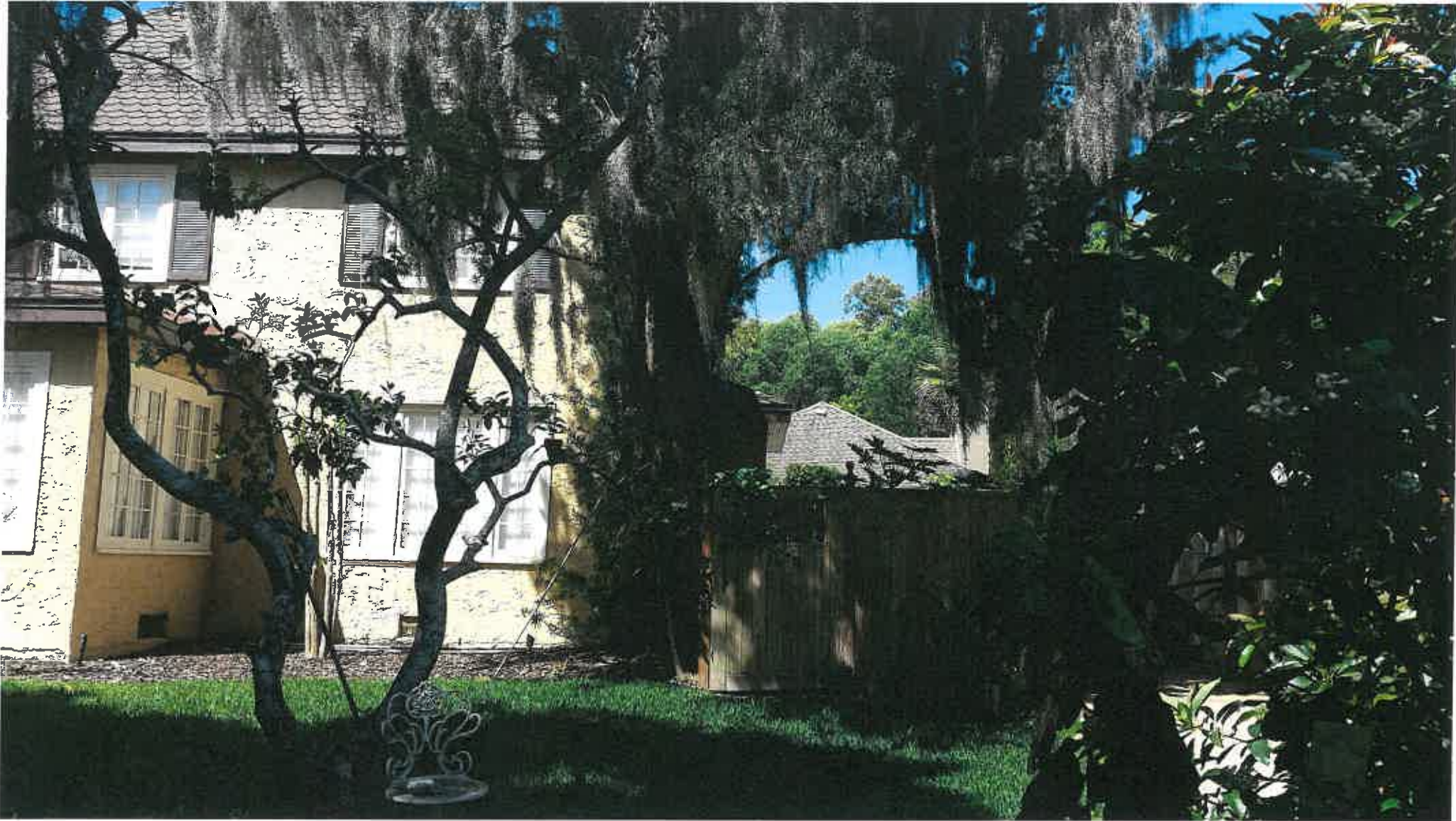
EAST SIDE ELEVATION REAR CORNER
