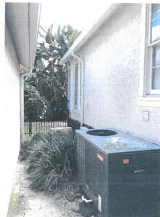
Existing House: view from East (rear yard)
