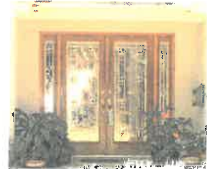
Inappropriate door proportion
