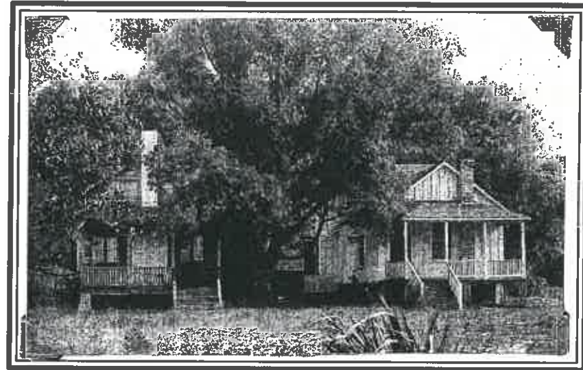
HISTORICAL PHOTO: VIEW FROM SOUTH
