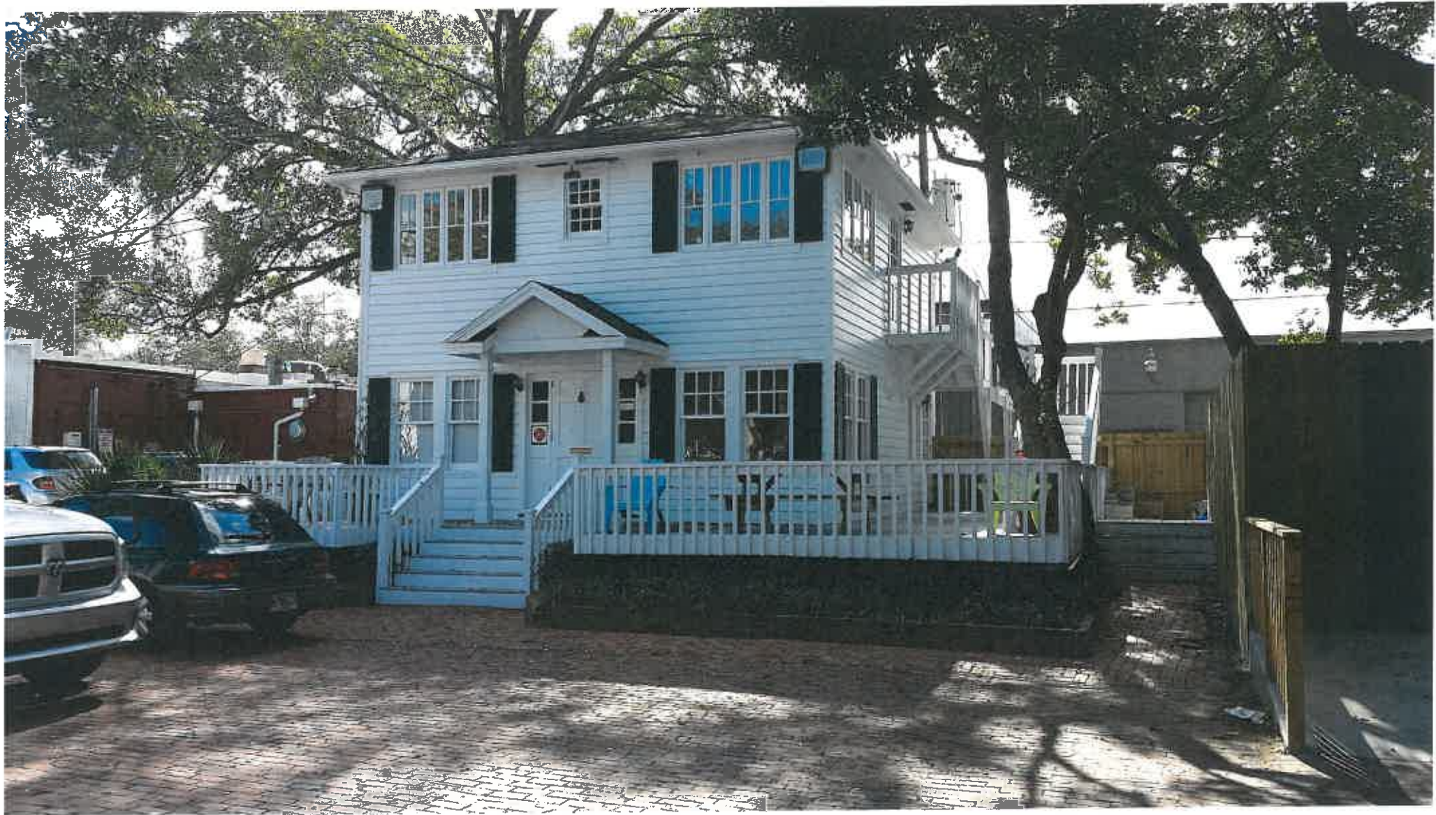
FACADE PROPOSED BUILDING WOULD BE TO THE RIGHT OF PHOTO
