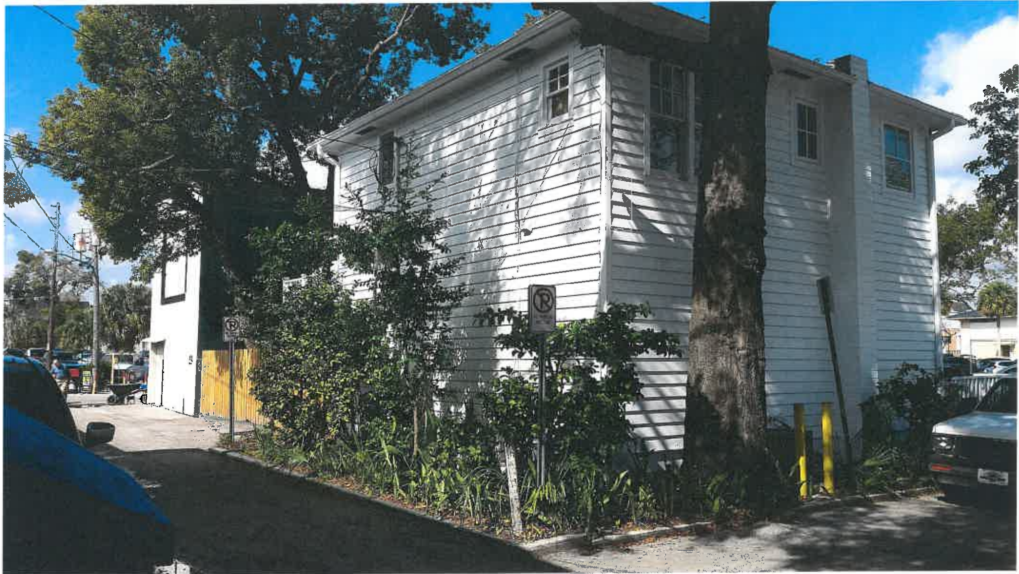
REAR & EAST SIDE ELEVATION LOOKING WEST
