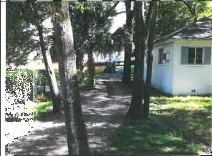
Example 2 of vehicular traffic on Rollins constructed roadway.
