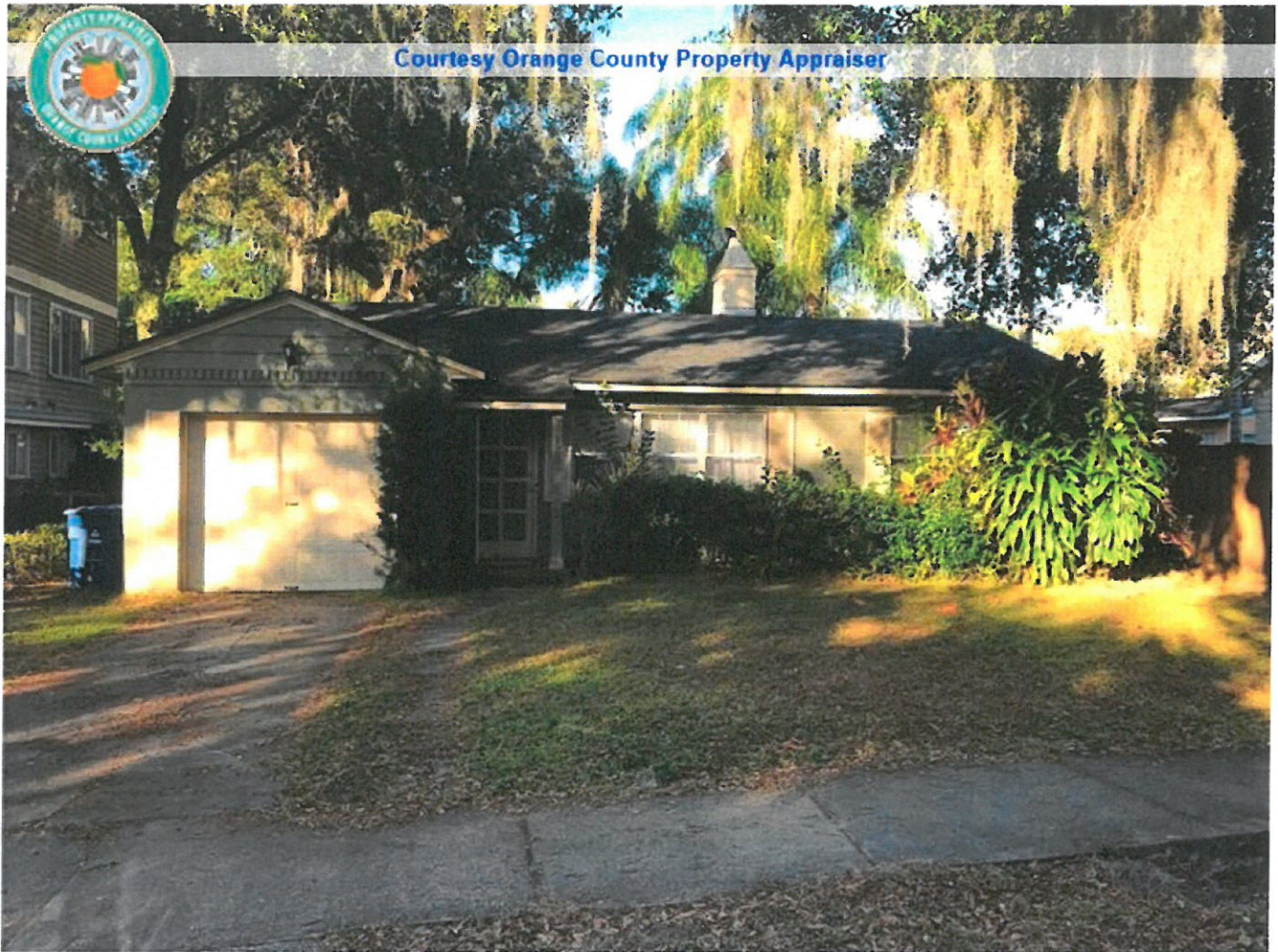
723 MARYLAND AVE, WINTER PARK, FL 32789 12/28/2020 8:49 AM
