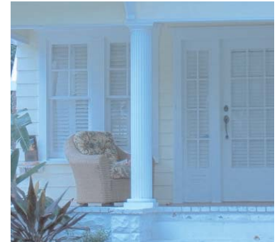
Replacement column not consistent with building style
