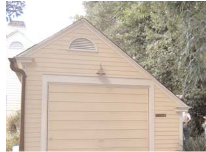
Roof shape not consistent with district
