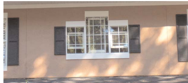
Inappropriate Window Type
