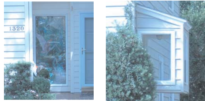
Examples of inappropriate window additions
