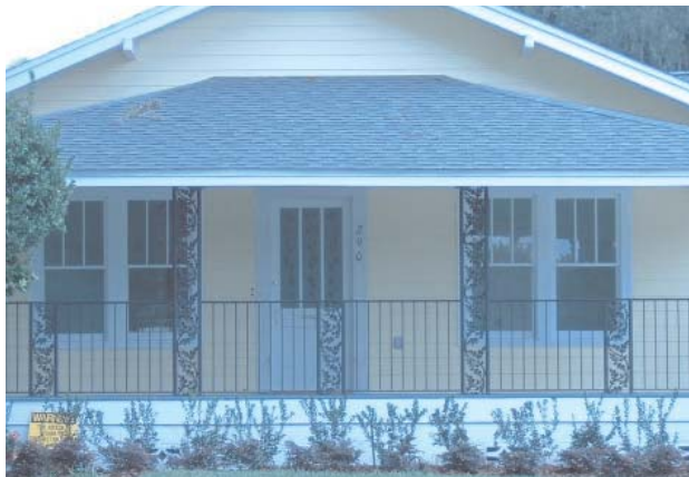
Porch supports not consistent with style
