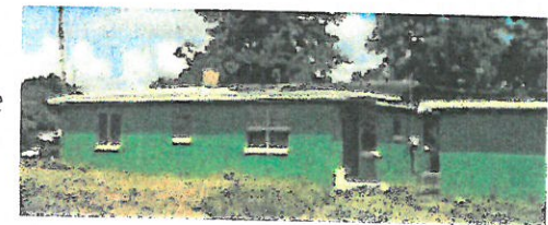
Inappropriate Colors for a Historic District
