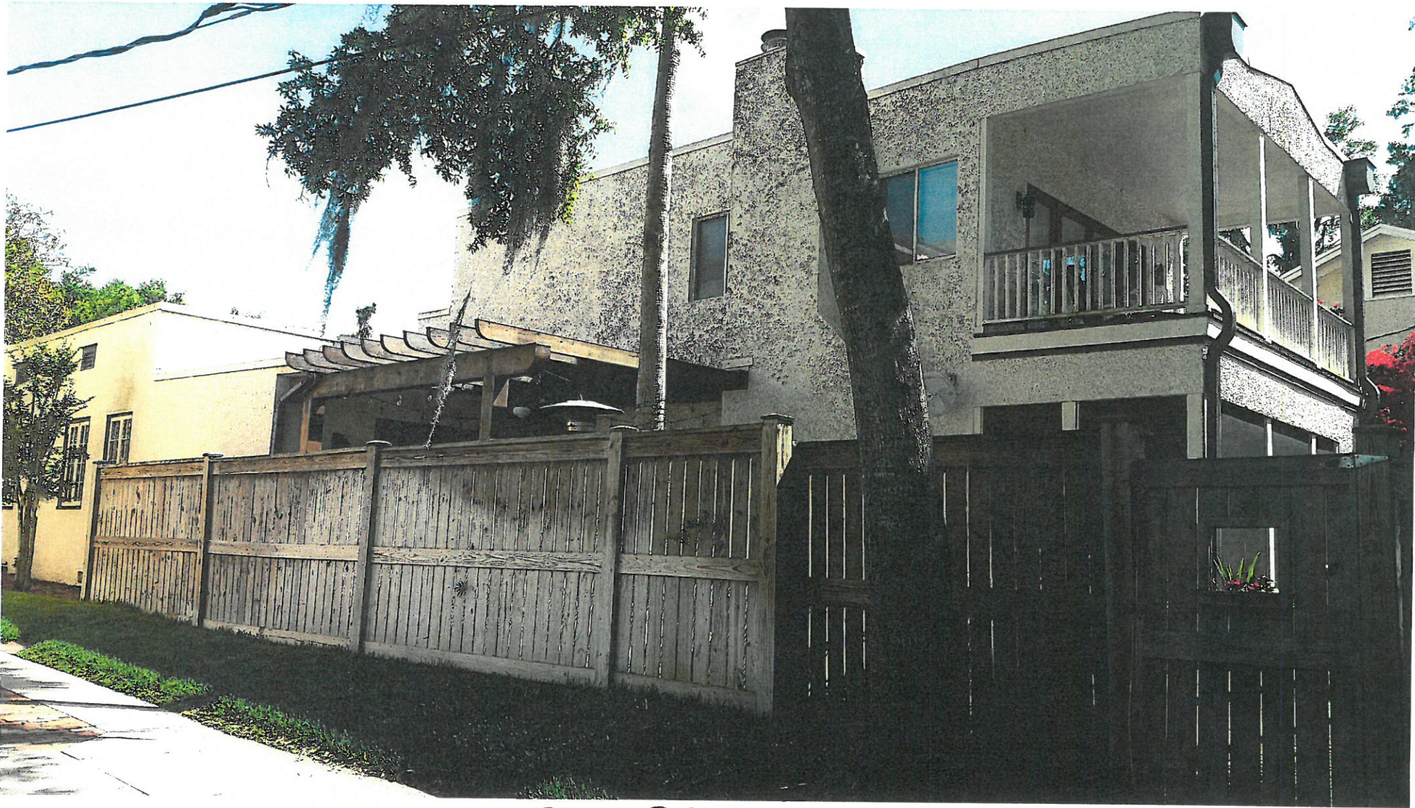
WEST SIDE ELEVATION FROM REAR
