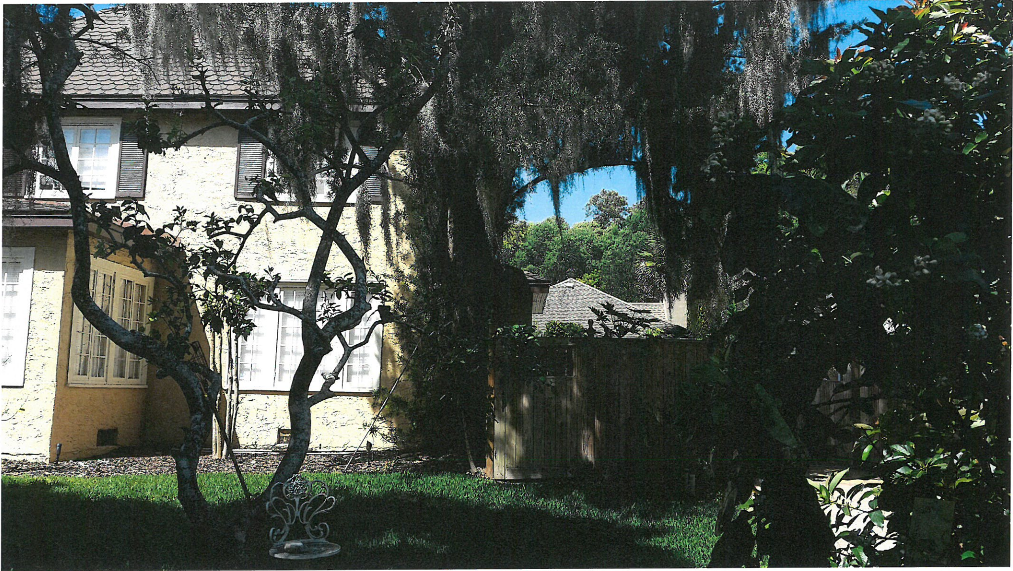
EAST SIDE ELEVATION REAR CORNER
