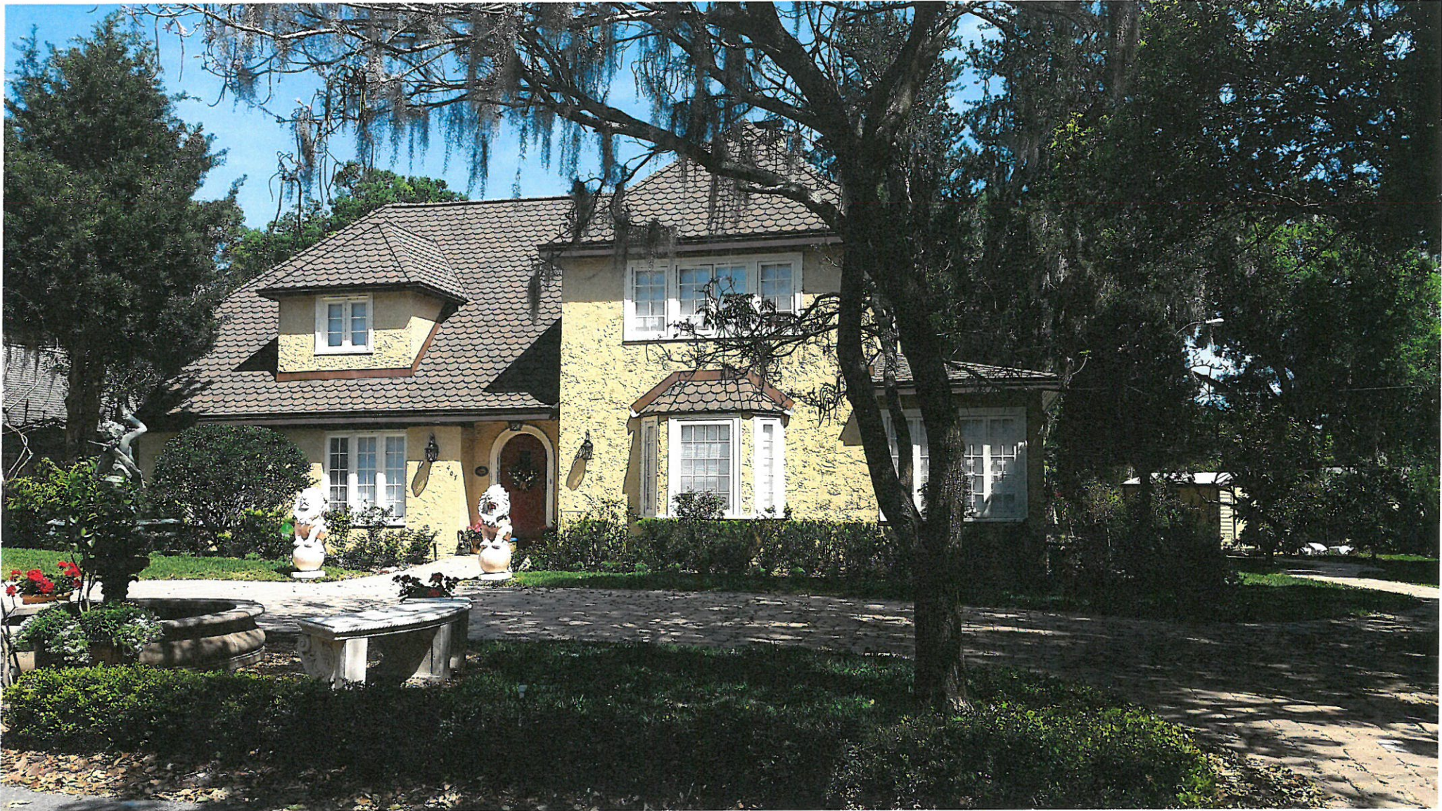
SOUTH FACING FRONT ELEVATION
