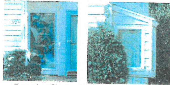
Examples of inappropriate window additions
