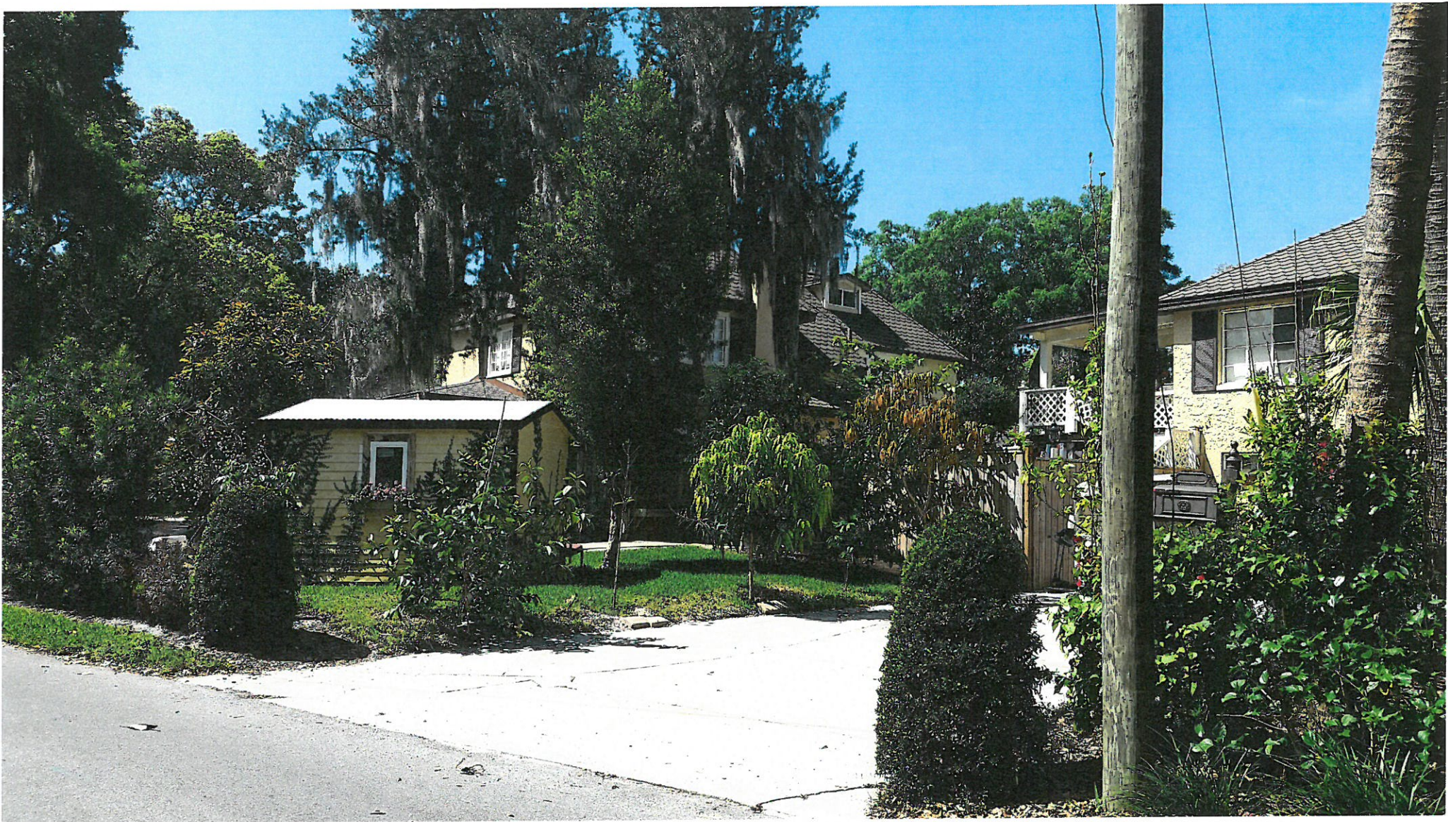
REAR ELEVATION & NORTHEAST CORNER VIEW FROM OXFORD ROAD
