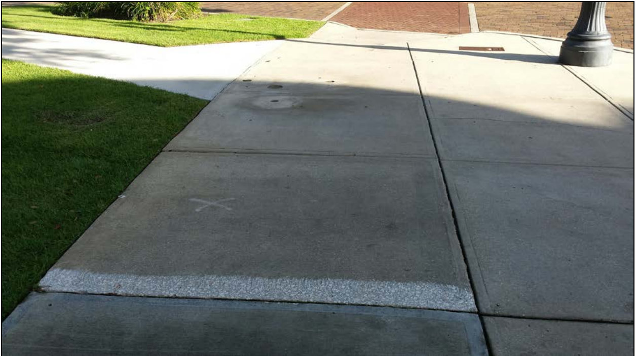
Park & Lyman ( southwest corner )
