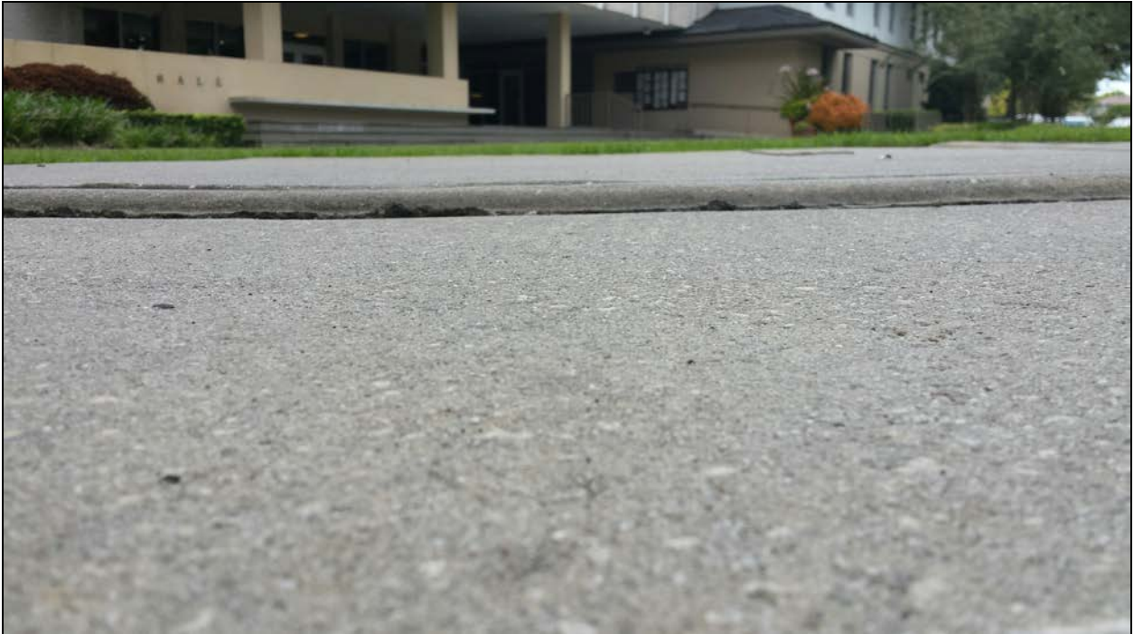
Park & Lyman ( southwest corner )
