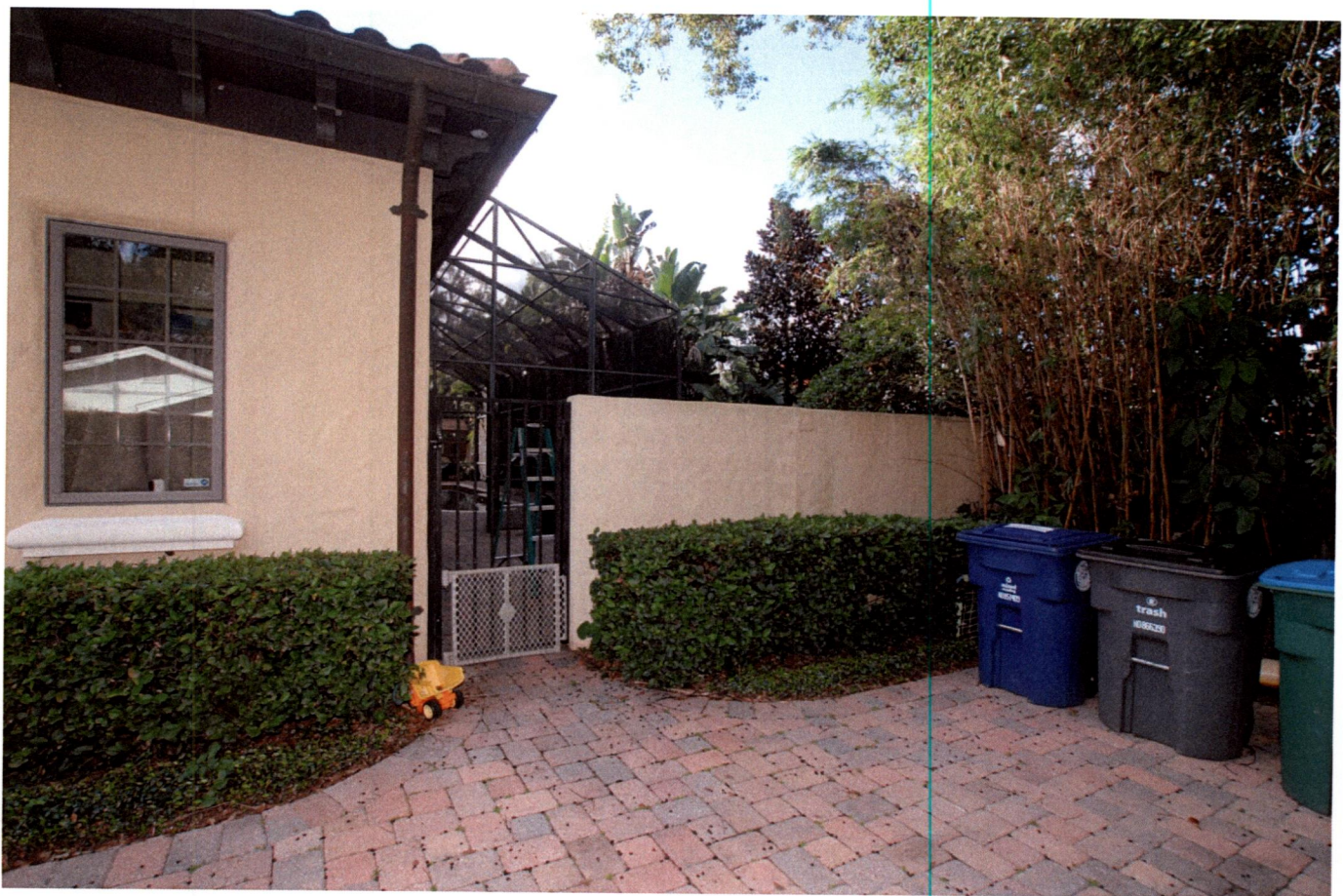
Side view from existing East Elevation
