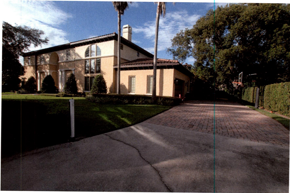
Front view from existing South Elevation (right side)
