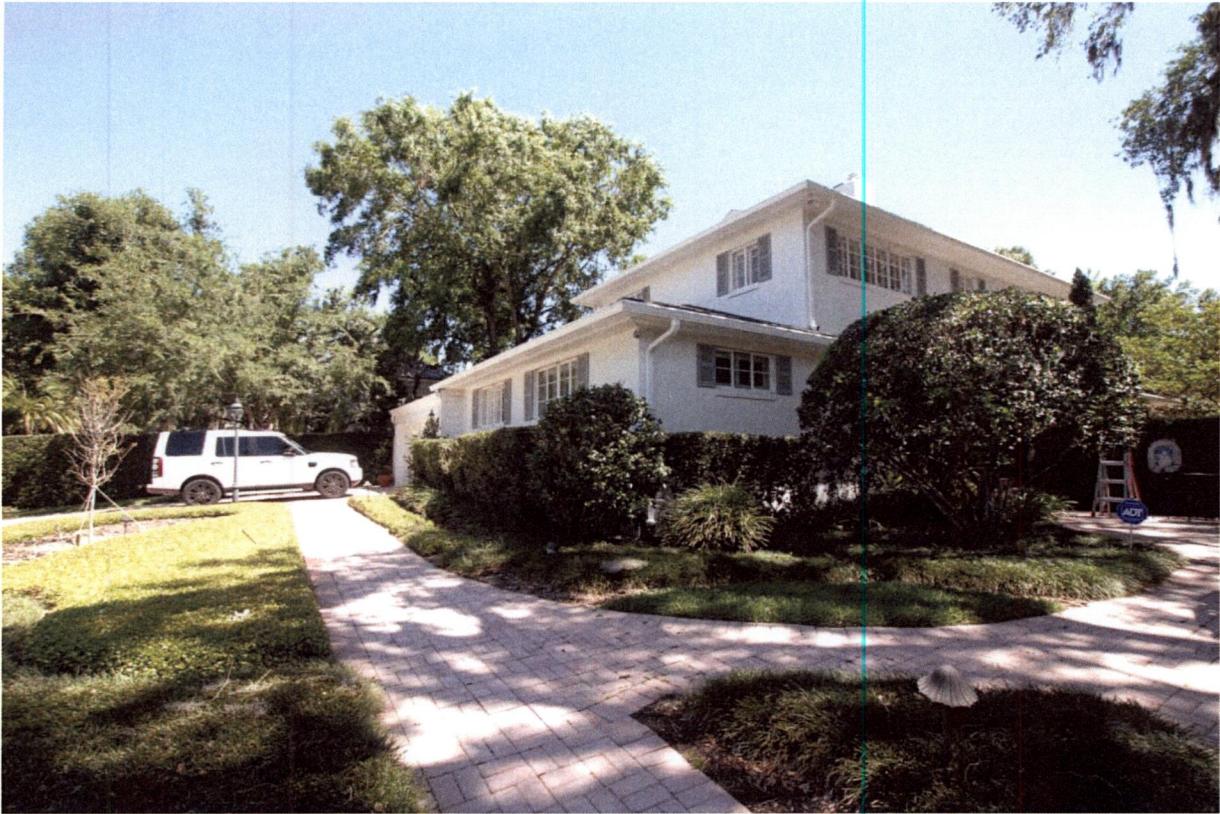
Front view from South existing elevation
