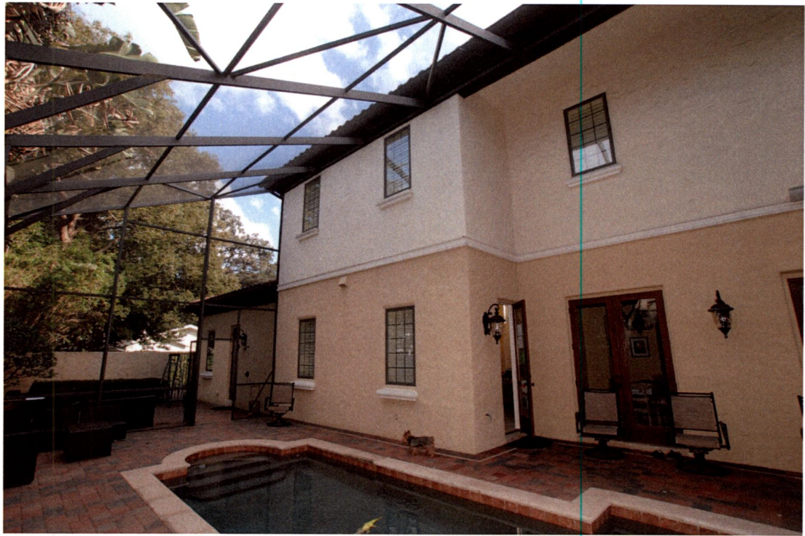
View of existing North Elevation (left side)
