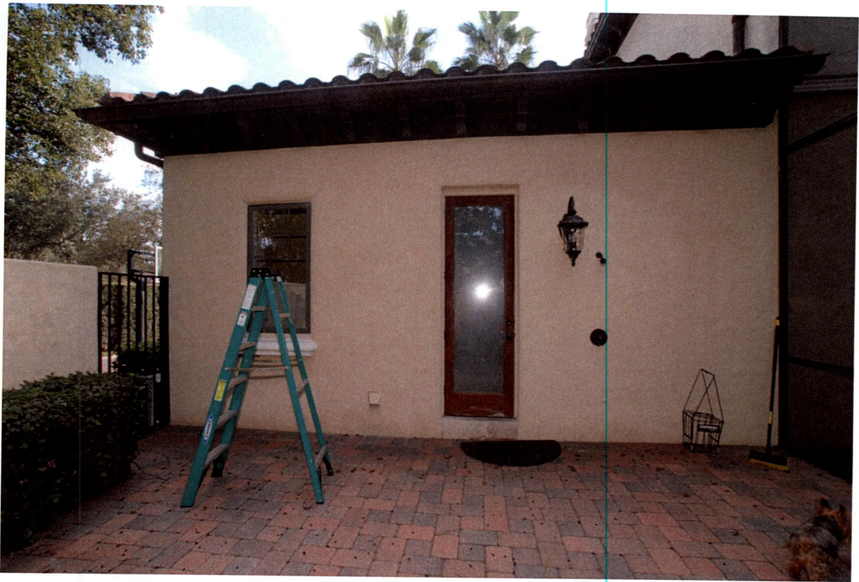
View of existing North Elevation (right side) (Area of Proposed Addition)
