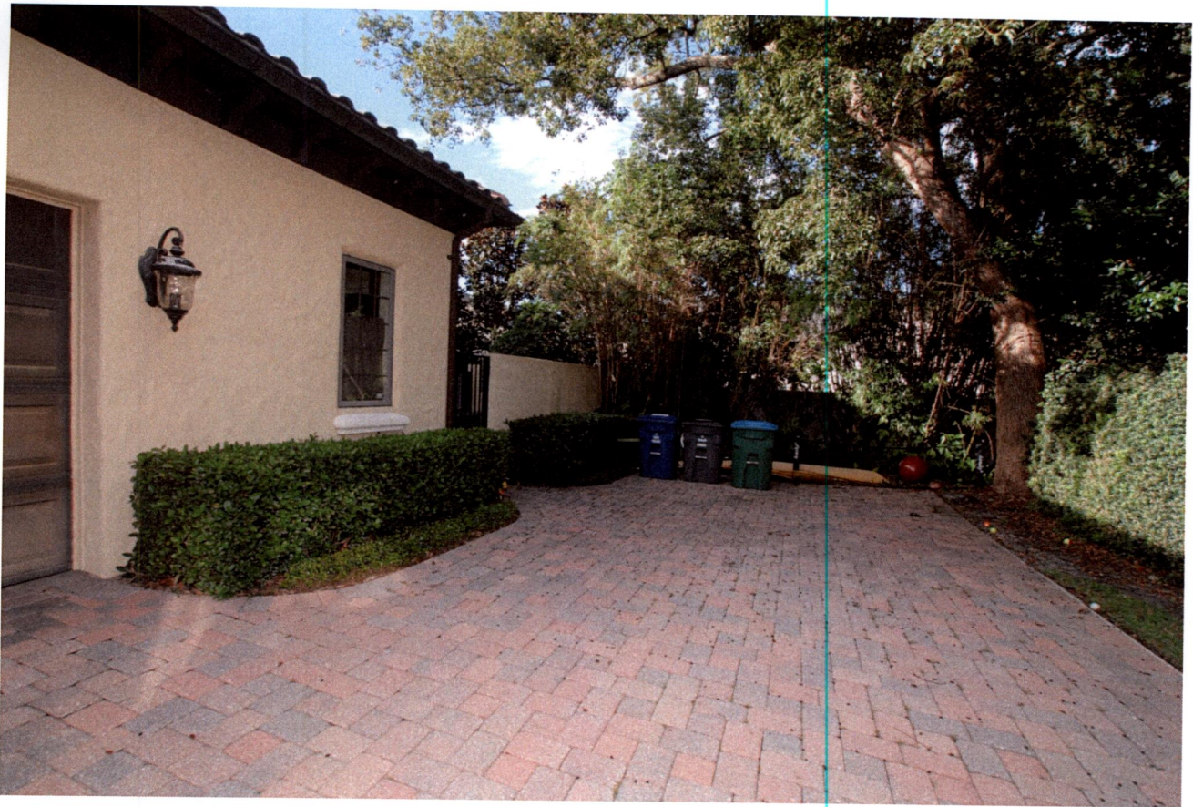
Side view from existing East Elevation
