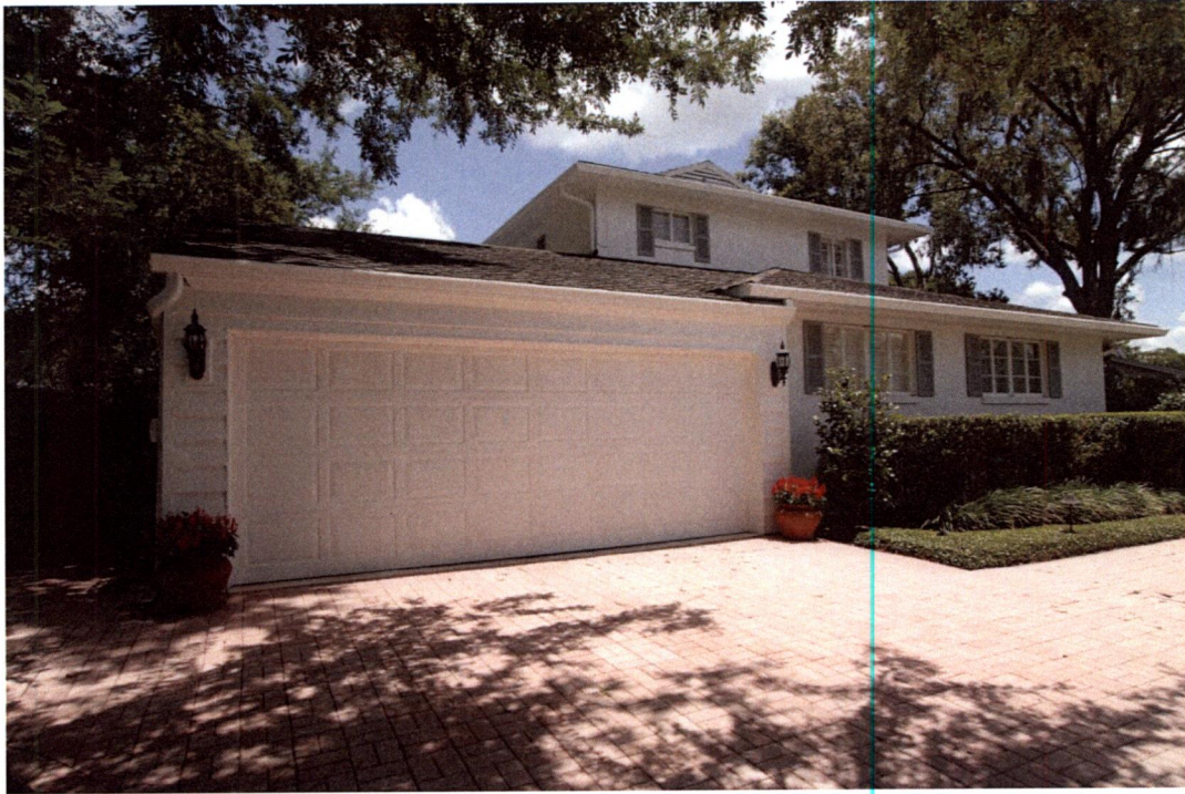
Front view from West existing elevation left side
