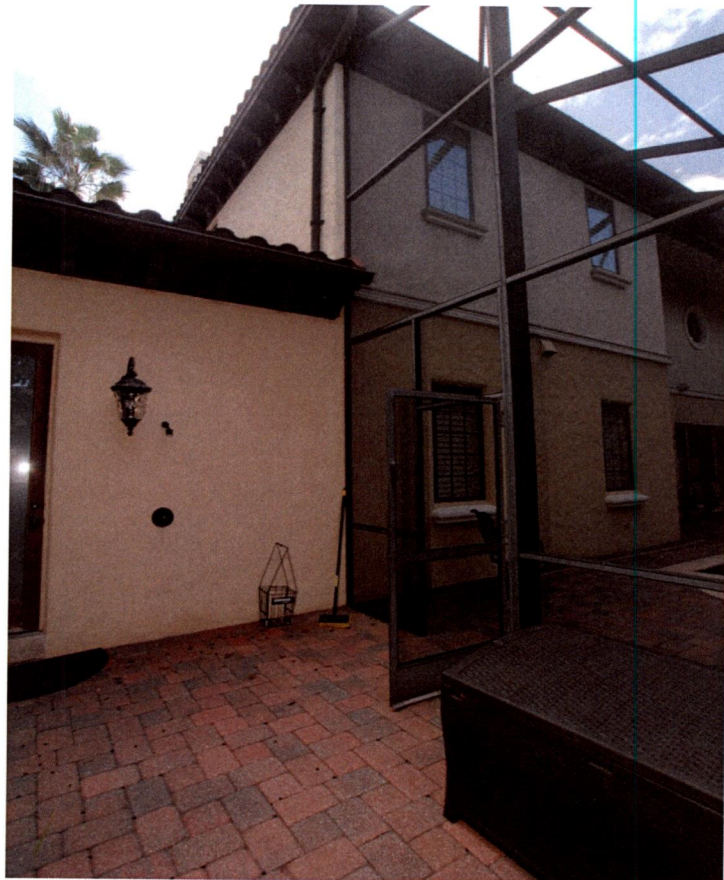
View of existing North Elevation (right side) (Area of Proposed Addition)
