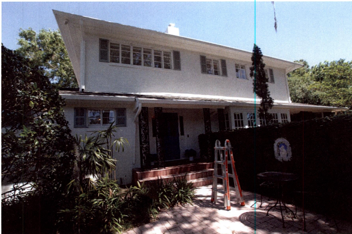
View from South existing elevation (Front Door)
