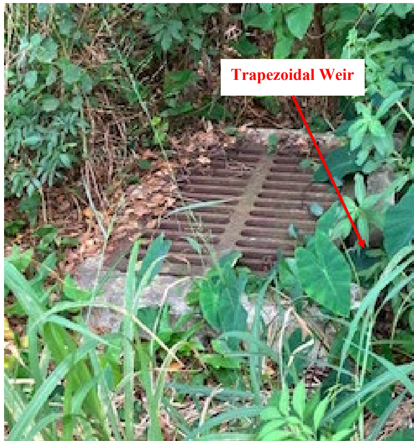
Photograph 10: Control Structure at Grove Street
