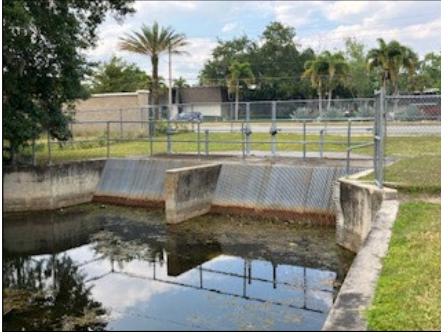
Photograph 1: Existing Lake Killarney Outfall
