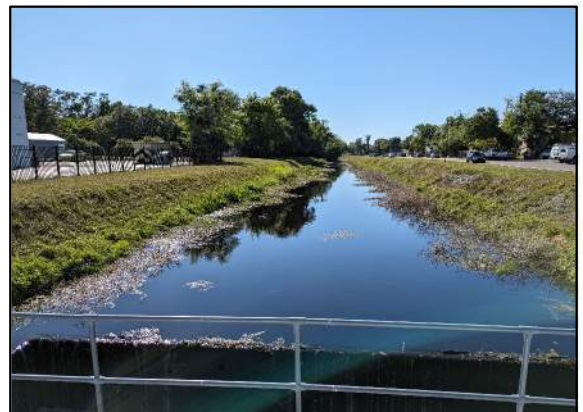
Existing Lake Corrine Outfall Canal (at Forsyth Rd)
