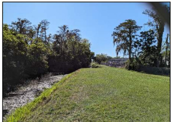
Existing Lake Corrine Outfall Canal (Looking West)
