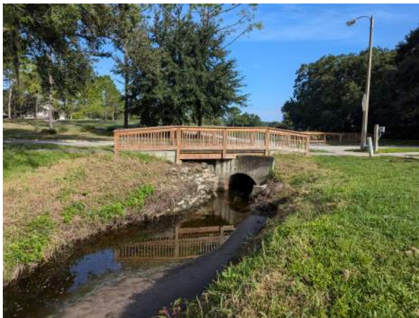
Golfside Dr – 72" CMP, Downstream
