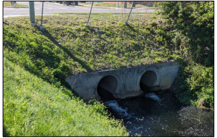
Existing Structure at Forsyth Road (Downstream)
