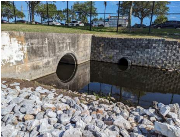
Baldwin Park St – Outfall Structure
