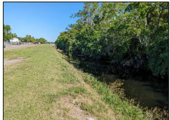
Existing Lake Corrine Outfall Canal (Looking East)
