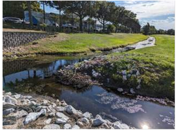
Baldwin Park St – Outfall Structure
