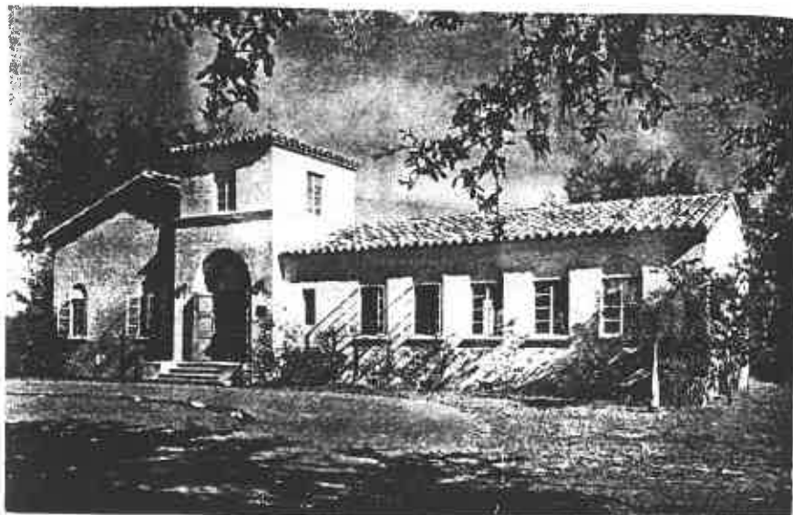
FIGURE 19. ROLLINS COLLEGE CHANGING ARCHITECTURE 1909-1940
