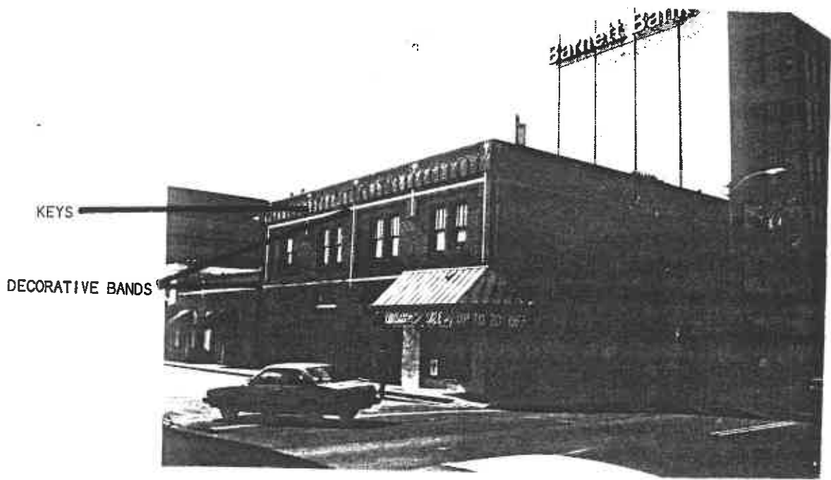
FIGURE 65. 206 SOUTH PARK AVENUE
