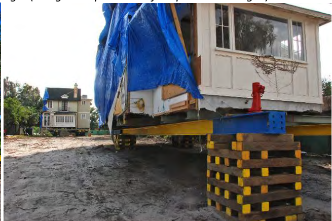
One-half of the Capen House delivered to the site and two halves to rejoin. (Images compliments of Stephen G. Pategas)
