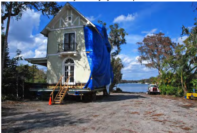
One-half of the Capen House delivered to the site and two halves to rejoin. (Images compliments of Stephen G. Pategas)
