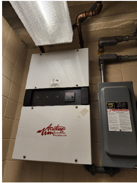
C-6: Tankless Water Heater
