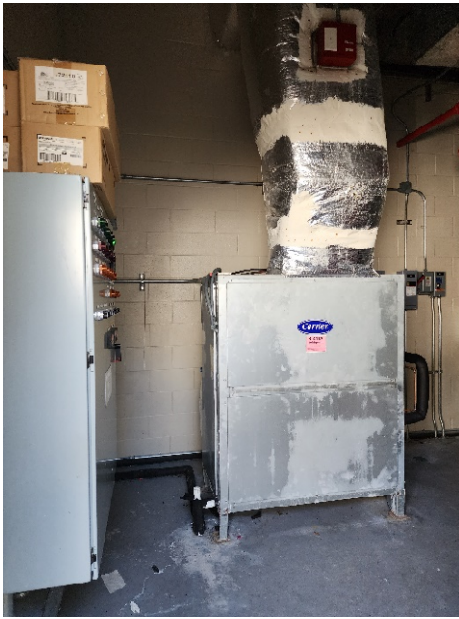
C-13: Carrier AHU
