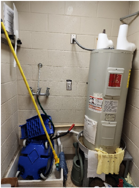
C-9: Electric Water Heater
