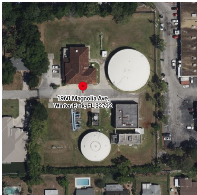
Figure 1: Aerial View of the Magnolia Plant Operations Building
