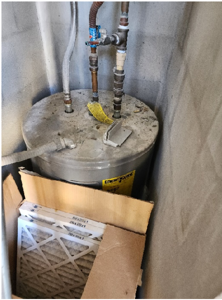
C-5: Electric Water Heater
