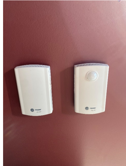
C-18: Temperature and CO2 Sensors
