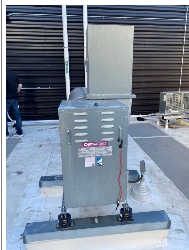
C-21: Exhaust Fan for Kitchen
