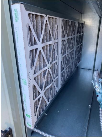
C-9: RTU Filter Detail
