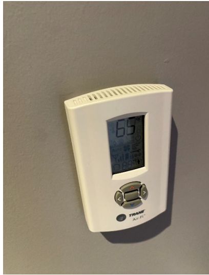
C-17: RTU Temperature Sensor/Thermostat
