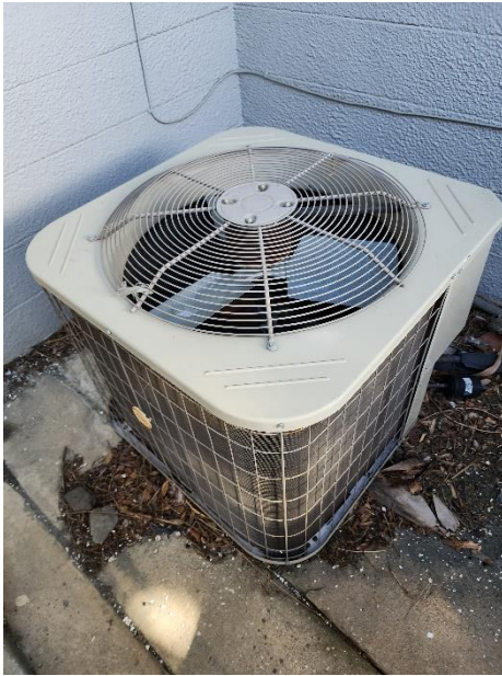
C-1: Condensing Unit (Photo 1)
