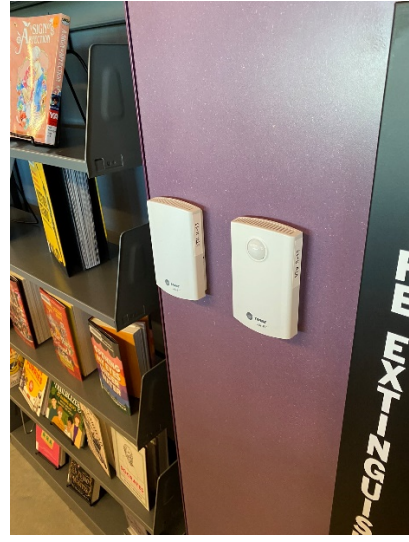
C-18: VTU-3-13 Temperature and CO2 Sensors
