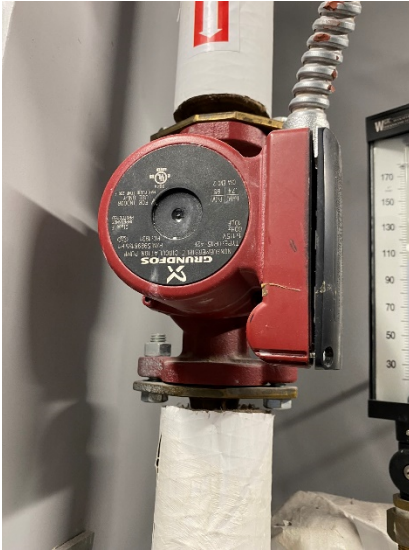
C-21: Hot Water Recirculation Pump
