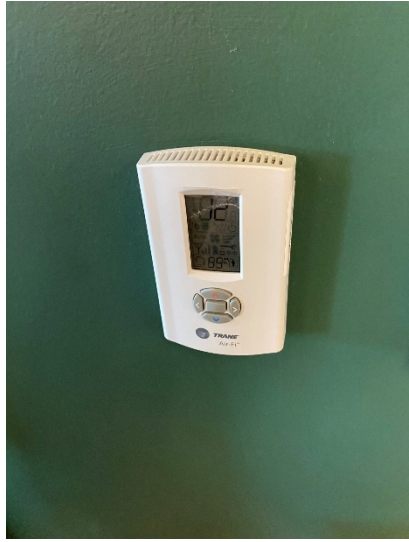
C-17: Level 2 VAV Temperature Sensor/Thermostat
