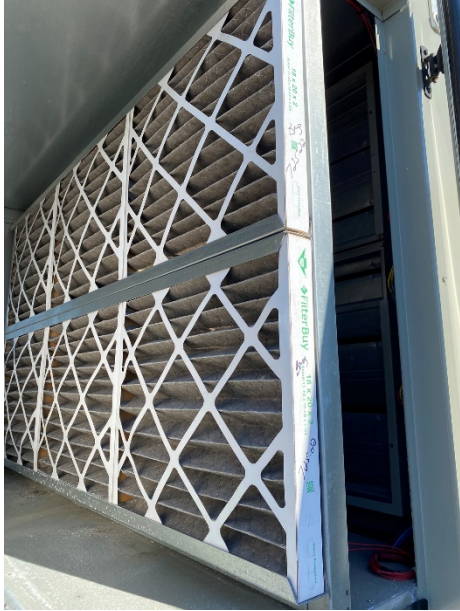
C-9: RTU Filter Detail
