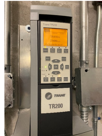
C-4: AHU-2 Outside Air Fan VFD at 100%
