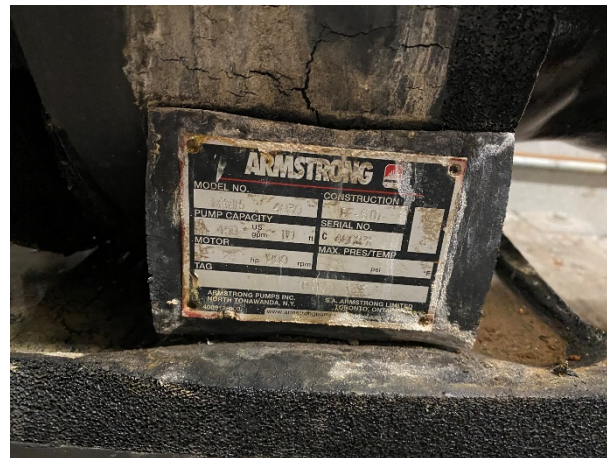
C-18: Chilled Water Pump Nameplate
