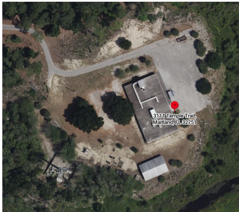
Figure 1: Aerial View of the Police Training Firing Range
