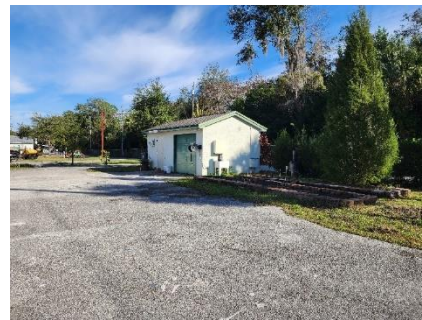
C8: Exterior of Building
