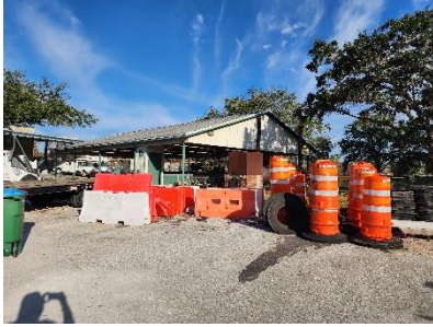
C30: Covered Storage Building
