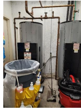
C20: Electric Water Heaters
