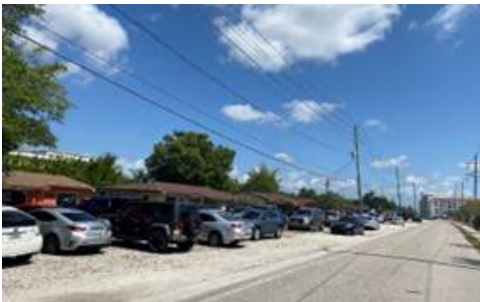
Defective street and parking layout. Cars parking on street frontage, continuous curb-cut.
