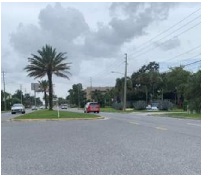
Over 1 mile of 4+ vehicle lanes to cross with no mid-block pedestrian signals, crosswalks, or points of refuge.
