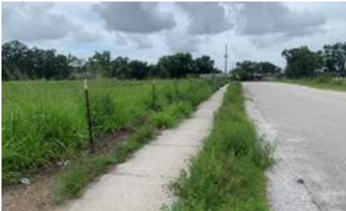
Defective street layout. Sidewalks and roadway serving large undeveloped, superblock, parcels near Ravaudage.
