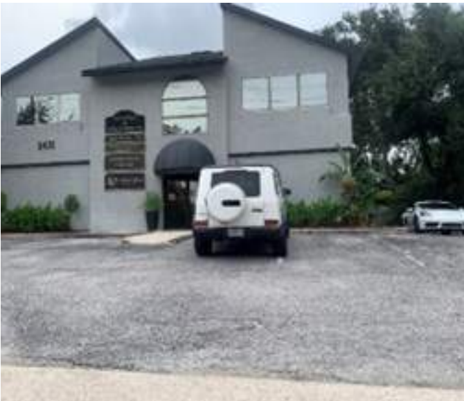
Faulty lot layout. Frontage parking directly off Lee Road. Traffic crosses sidewalk accessibility.
