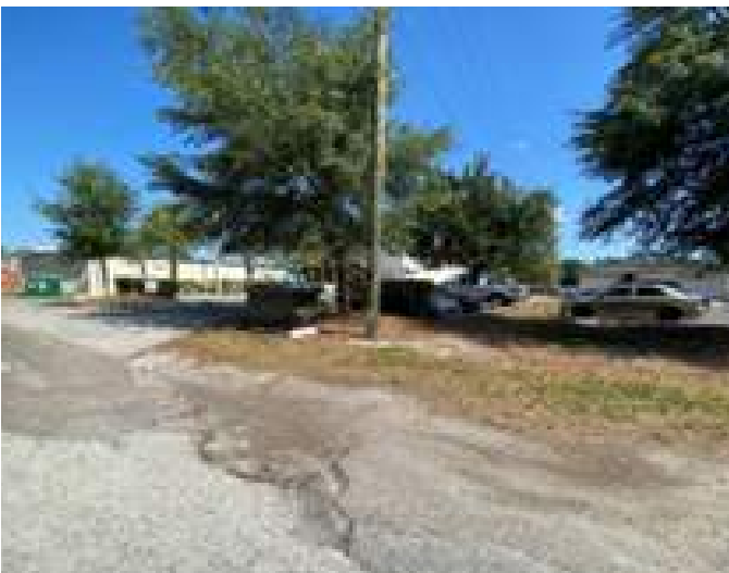
Deteriorated roadway surfaces.
