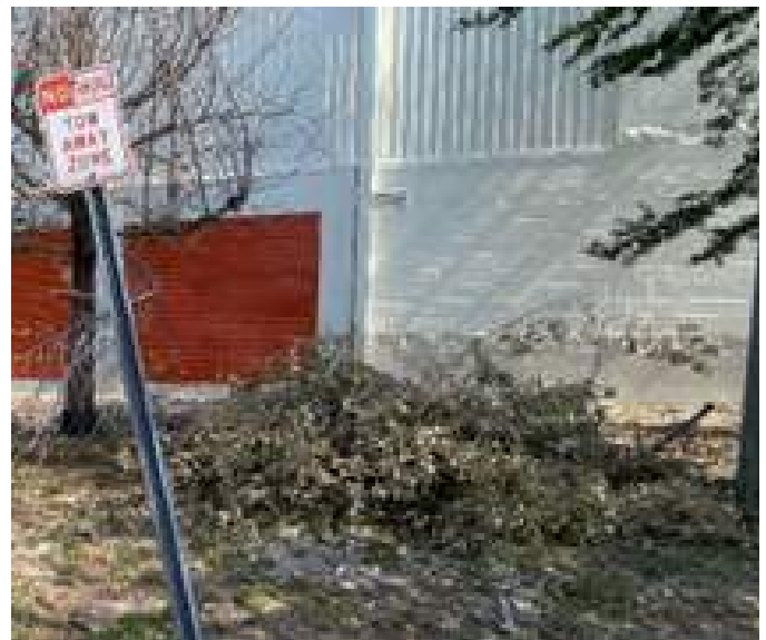
Unsafe and unsanitary conditions from illegal dumping at various location within the Fairbanks Avenue FON Study Area.
