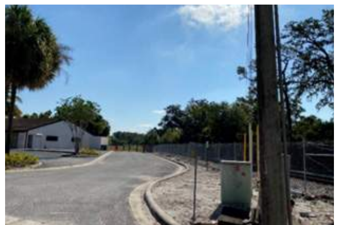
Disjointed and defective roadway layout within the Orlando Avenue Commercial Corridor FON Study Area.
