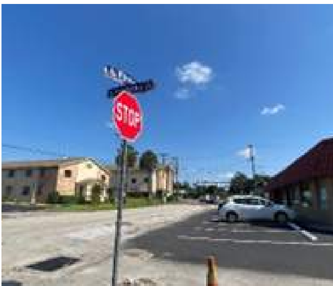
Church/School with no sidewalk accessibility. Parking configuration on commercial lot is unsafe.
