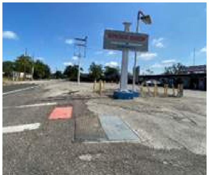
Convenience store with no clear sidewalk accessibility. Lot configuration prevents maximum use of site.
