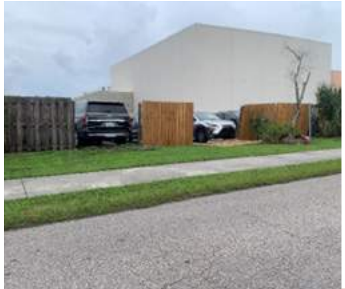
Deteriorated improvements boundary fence.
