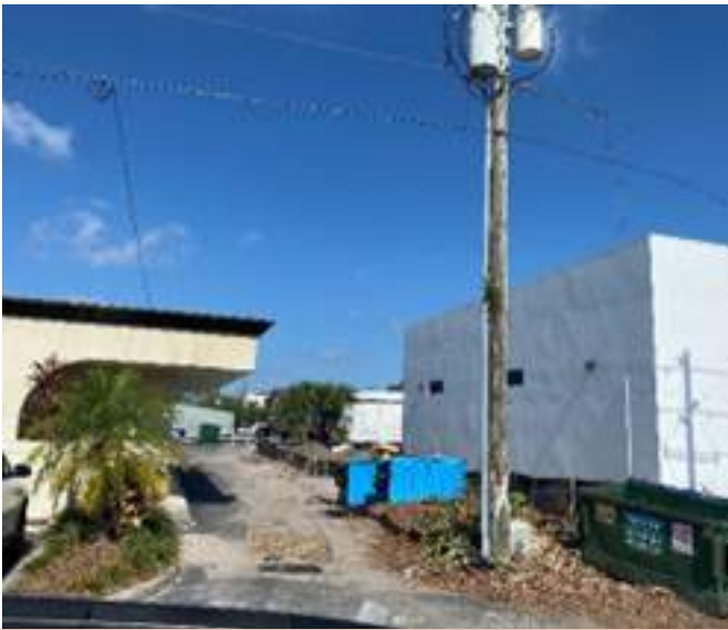
Lot configuration and accessibility affecting adjacent building set-backs, and screening of dumpsters.
