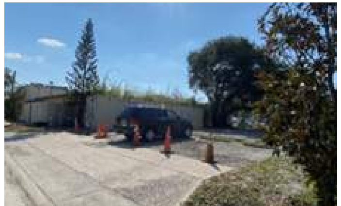
Inadequate and defective parking facilities within the Orlando Avenue Commercial Corridor FON Study Area.
