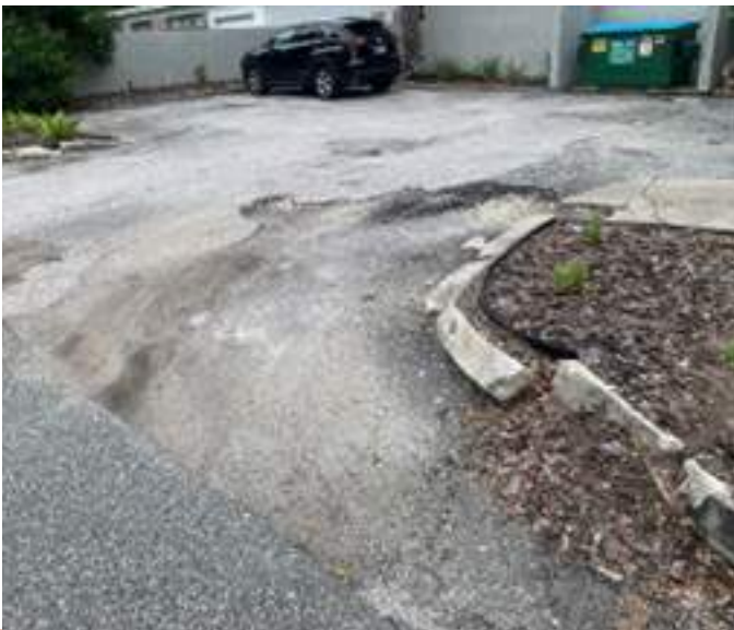
Deteriorated parking lot entry apron and curb.
